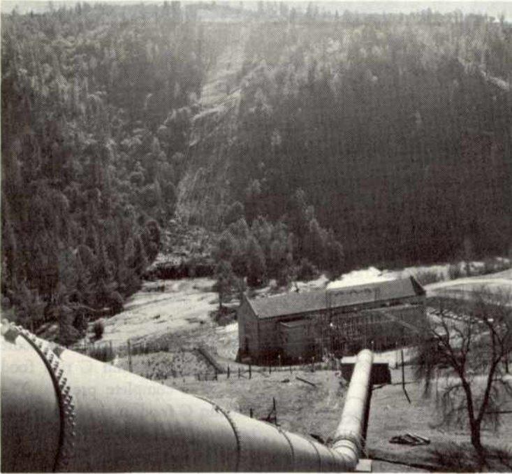
1. Morning becomes Electra, shown at the foot of the penstock on the left bank of the Mokelumne in the heart of the Mother Lode. Transmission lines carrying Electra's generation into the rest of the PG&E system can be seen in the background on the other side of the river.
