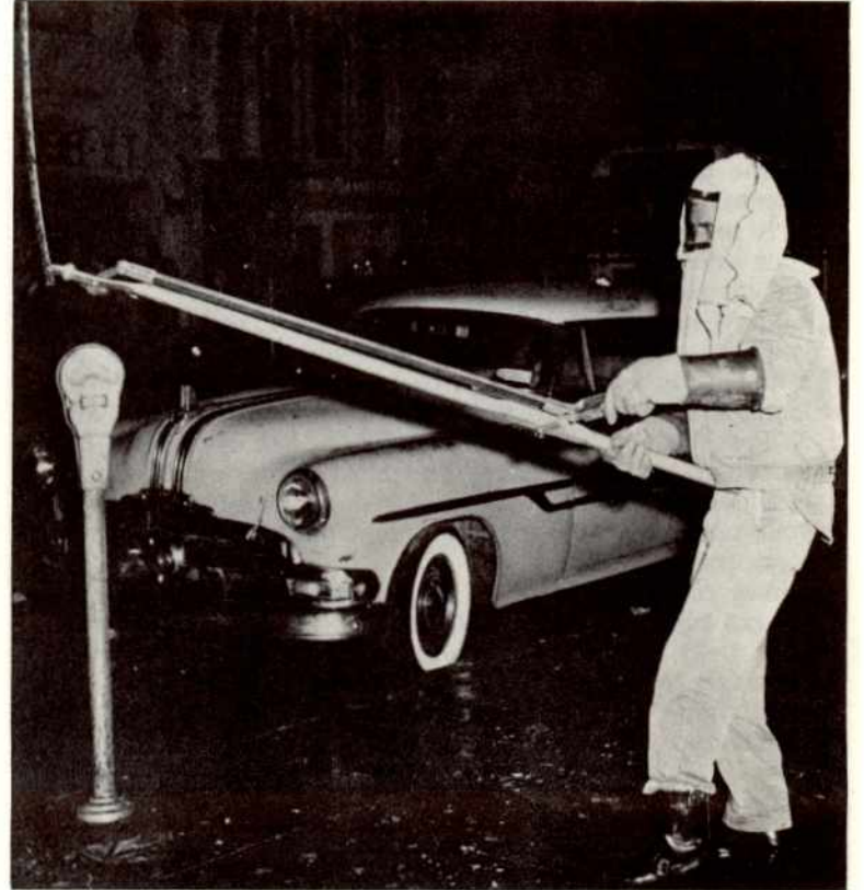
Troublemaker John Pickens shows how he cut the hot conductor in the clear on busy Fillmore St. in San Francisco. (Photo by John McBride of the San Francisco Chronicle.)
