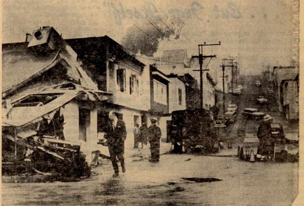
The morning after, the gas explosion scene near the Alemany offramp of the Bayshore freeway looked like this. The wreckage of Mr. and Mrs. Toy's house is shown above. In the picture below, the gas line which feeds Hunter's Point power plant is shown. The handkerchief marks the point of explosion and the repairs. At lower left, gas men, who relieved crews who worked most of the night, continue work at the scene.
