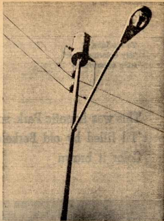
The old and the new—found on adjacent poles. The new steel pole with the transformer mounted above represents a compromise between unsightly overhead and more expensive underground distribution.
