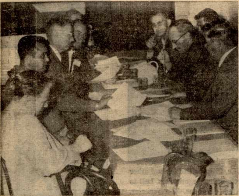
Steward Fountain indicates a point to Tony Boker as the rest of the General Construction caucus looks on. From left to right: Joe Mayes, John Roman Jr., Lester Price, John Scheeringa, William Barrett, Belden Trigg, Cliff Andrews, Tony and Steward.
