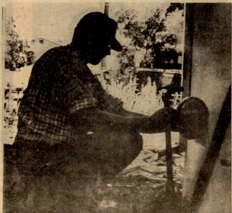
John Kowall, Apprentice Fitter, is installing a meter in this picture as one of the final steps in providing service to a new home in Stockton.
