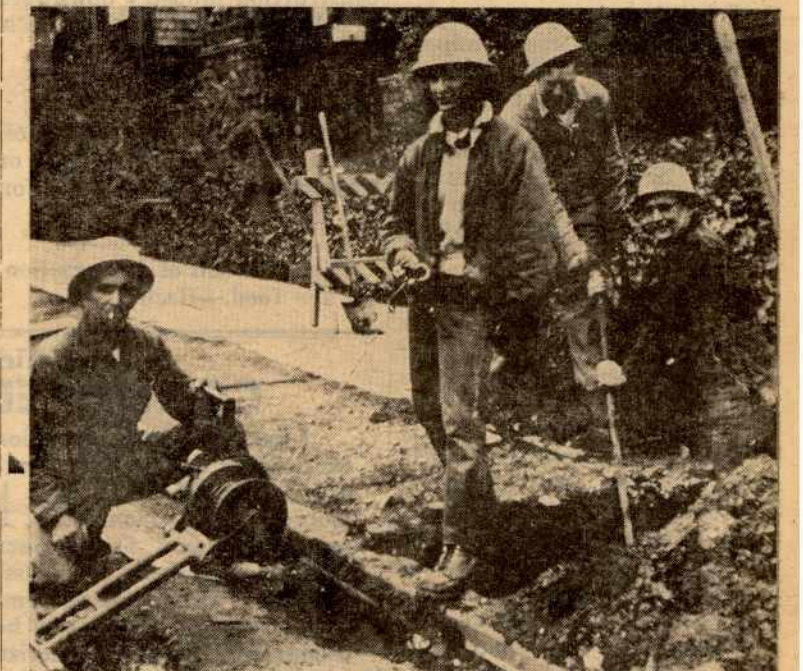
Good news to General Construction Department members has been the large amount of Gas Construction work in the East Bay Division. Pictured here on reconstruction work due to the resurfacing of Woolsey Street in Berkeley are L. to R., Leon Gilbert, Steve Yabara, Harold Cantrell, and Shop Steward Walter Henderson.
