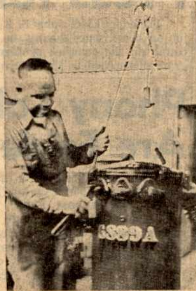
Charles Bagley, Transformer Repairman, working on Transformer at San Rafael.
