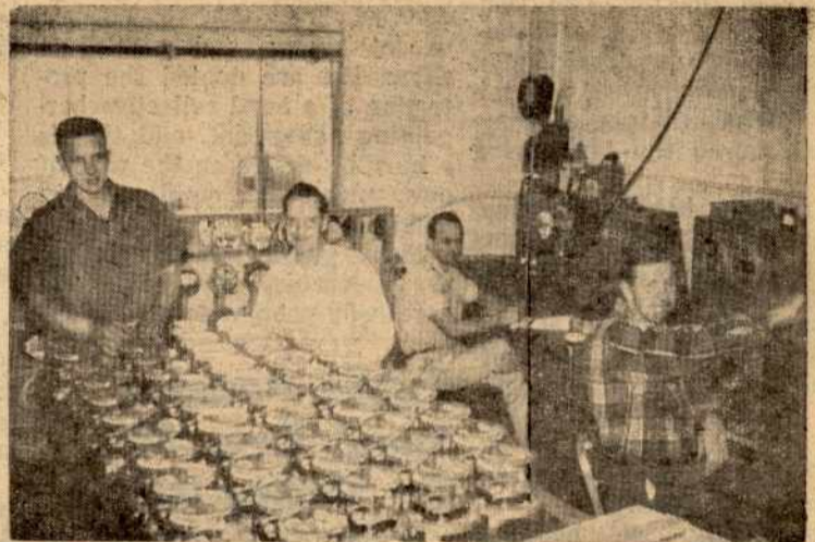
Shown at Meter Test Bench Section at Reno Electric Meter Shop where meters are tested, repaired and returned to service, are, left to right, John Gisclone, part-time employee and college student, and Local 1245 members Norman Harris, Meter Clerk and Shop Steward; Gene Thraikill, Meterman; and Reno Unit Chairman George MacDonald, Meterman.
