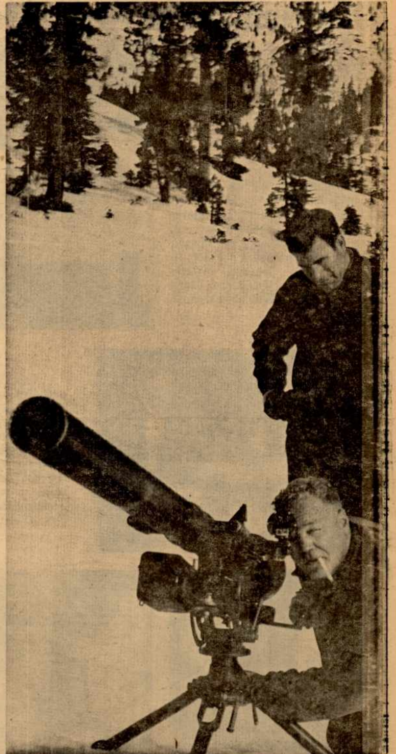
BOOM! DOWN SHE COMES! That's Monty Atwater, US Forest Service snow control specialists, aiming a 75 mm recoilless rifle at a potential avalanche. John Mortizia, lift manager for the Squaw Valley Lodge, looks on. The idea is to detect a potential avalanche and to cause it to slide down by shooting into it. This is one part of a safety program at Squaw Valley to keep slopes safe for skiers.
