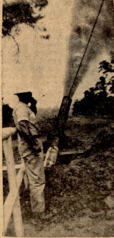
Flame thrower? Nope! It's the purge stack on the new 145-mile, 12-inch Gas main between Red Bluff and Fortuna. "Purging a line" is the blowing out of all dirt and foreign material with air under extremely high pressure, followed by Gas, also under high pressure to assure that the main is completely filled with Gas, leaving no air pockets in the line. Completion of this job brings Gas, for the first time, into Eureka and more jobs for more Gas Workers in this area.
