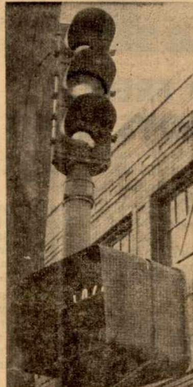
Vehicle and pedestrian traffic signal at a downtown intersection. Although an irritant when you always seem to "hit them on the red", imagine the mess if they weren't there.
