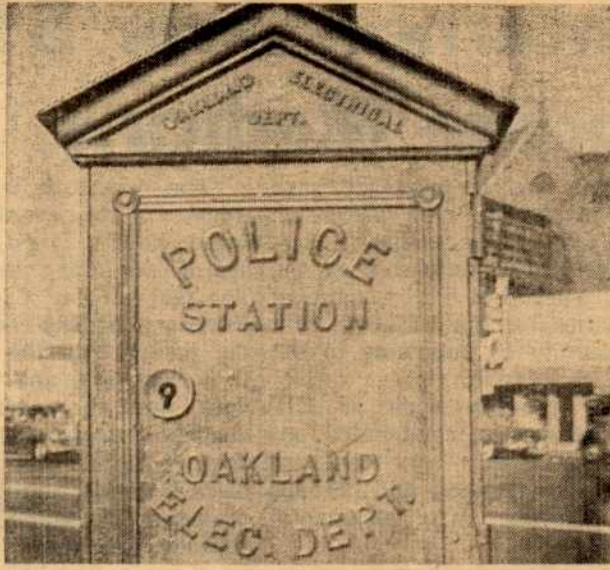
Just one of the 300 or more Police Call Boxes which our City of Oakland's Electrical Dept., must keep in top working condition for the protection of the 1/2 million or so Oakland residents.
