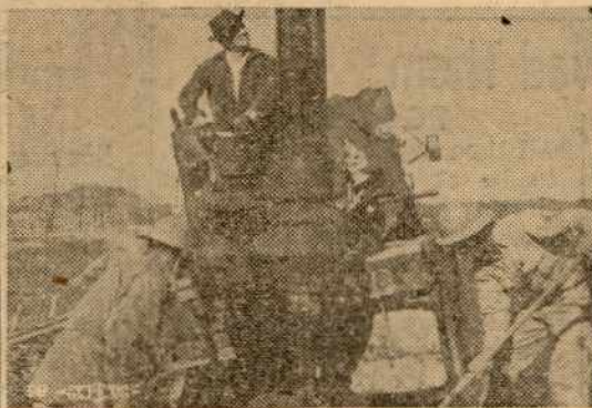
Pole holes now are dug by machine, although the old shovel is still a necessary tool.
