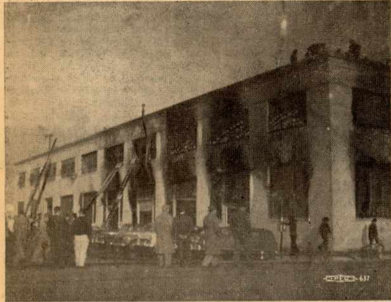
Above picture taken about an hour after the explosion, shows the terrific heat and force generated and its effect on the building. The blast occurred downstairs in corner of building nearest the camera, forcing gas upstairs where it ignited and gutted both floors and the roof.
