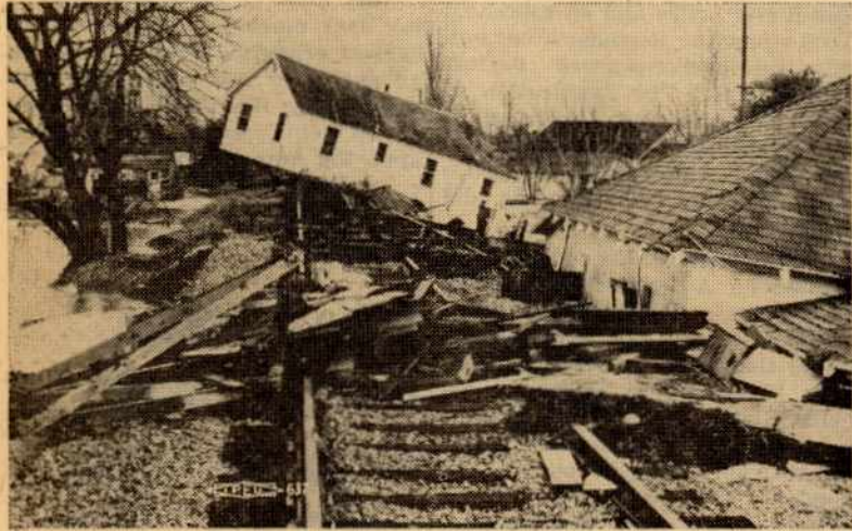
A house was tilted at a crazy angle on top of railroad tracks and another was buckled against the rail embankment as the flood waters receded in Yuba City. The wreckage as seen in the picture is indicative of the havoc left by the Christmas week inundation of a large section of Sutter County.
