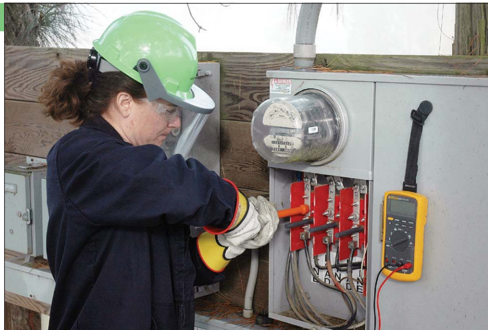
Stacy Wallace, a journeyman wireman for Wellington Energy, removes the old electric meter powering a rural residence in Sonoma County.
