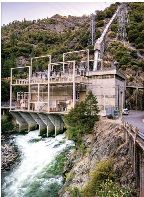
The Jaybird Powerhouse in Fresh Pond, Calif.
