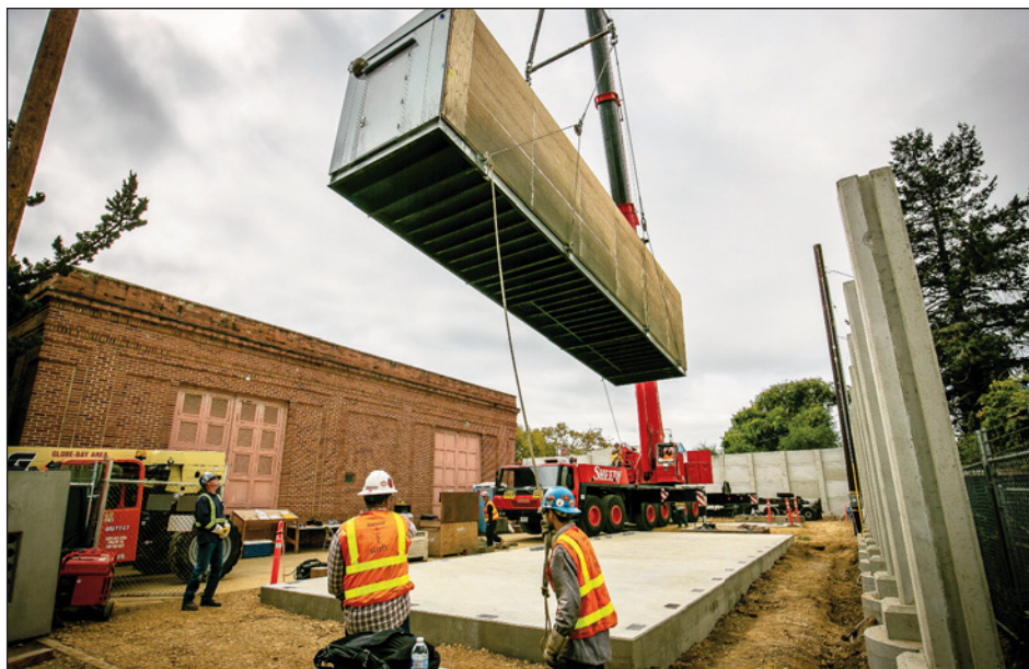
A 350-ft crane was used to set the new building at the sub.
