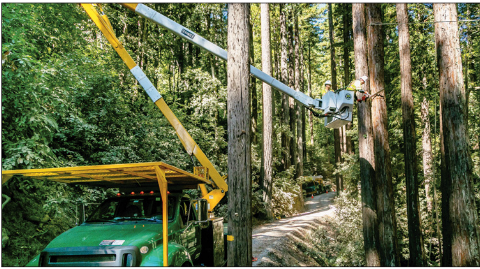
An IBEW 1245 crew with Davey Tree performs fuel reduction work in Boulder Creek, CA.
