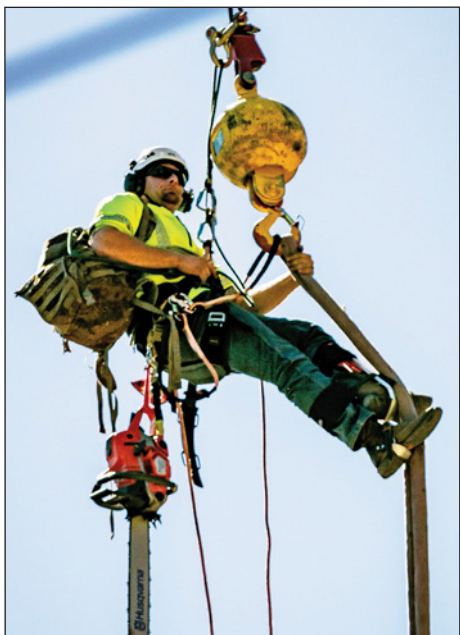
IBEW 1245 member Tyler Sterns from Arborworks rides a cable from a crane.
