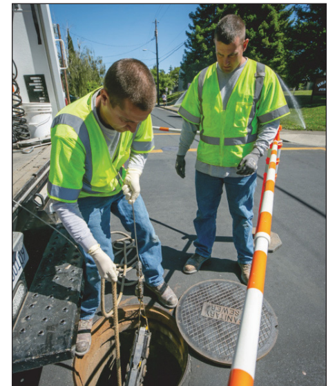
Chris Worlow and Ryan Alves put a camera into a sewer to do a visual survey.
