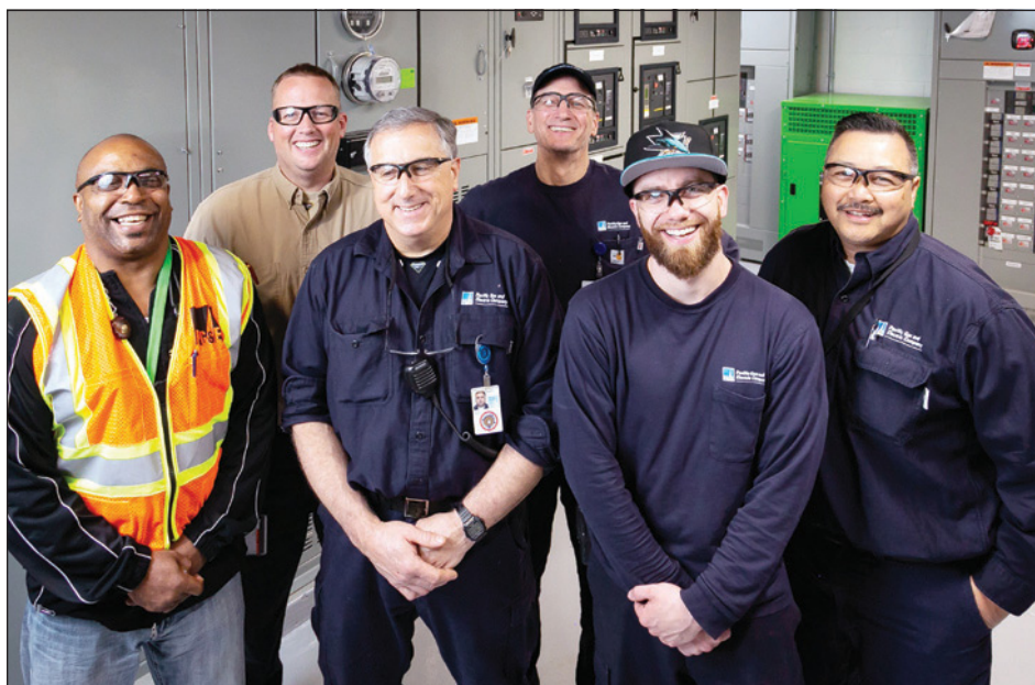
Facilities technicians (from left) Victor Givhan, Robert Sadler, John Saisi, Gary Maschio, Kevin Lavender, and Vince Almacen in the 2B switchgear room at 77 Beale
