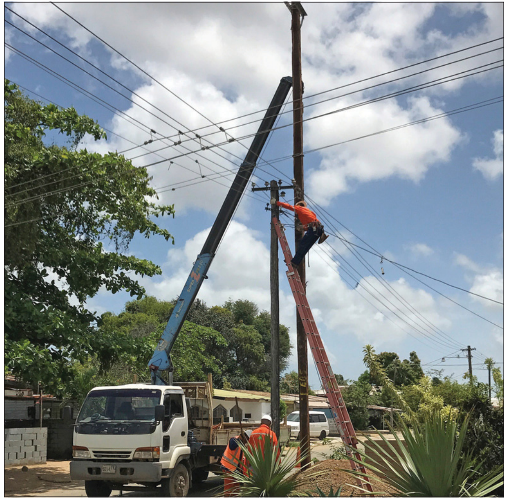
At a new business project to improve voltage, the SABI trainers were thrilled to see the Surinamese linemen implementing the safety standards they were taught, including high visibility vests, traffic control with road cones, three-way communication, bucket harness, tying off ladders, and grounding the primary and isolating secondary from back feed.
