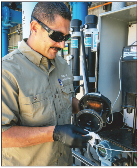
Jorge Valencia cleans the turbidity meters at the reclamation plant.
