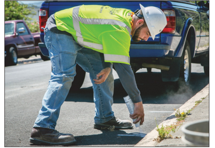
Eric Webb locates and marks the street for future work.
