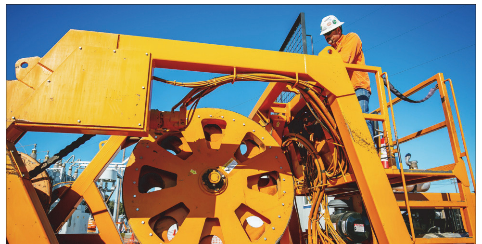
Tom Stansberry with Dacon on the cable puller
