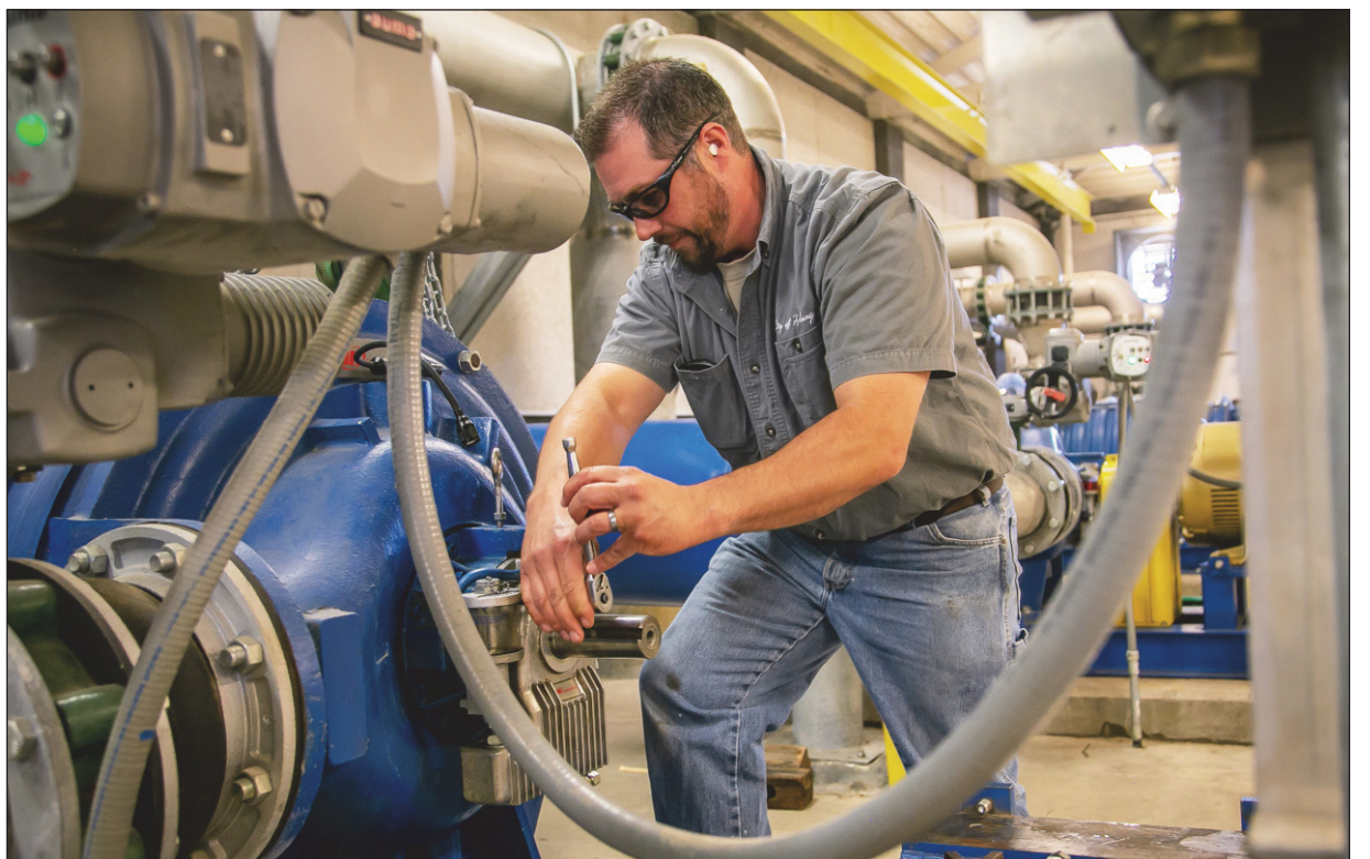
Mechanic Dustin Huse works on a pump at the reclamation plant.
