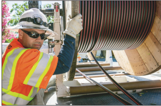
Lineman Jorge Hernandez pulls cable.
