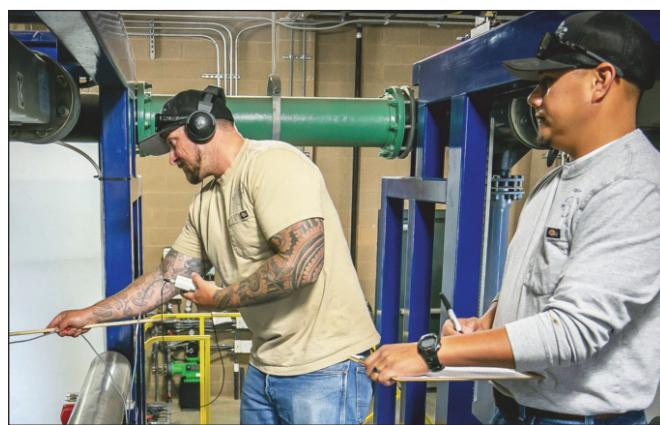
John Sanneman, (left), and Eddie Uribe test filters at the Water Micro-Filtration Plant.
