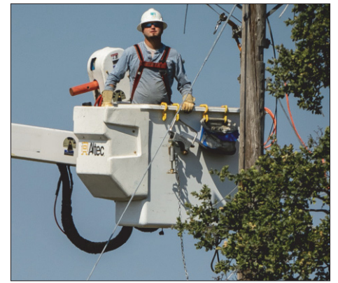
Casey Prine works in a bucket
