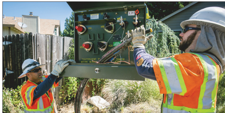
Lineman Jorge Hernandez, left, and Apprentice Linemen Chayton Osmon replace a box.
