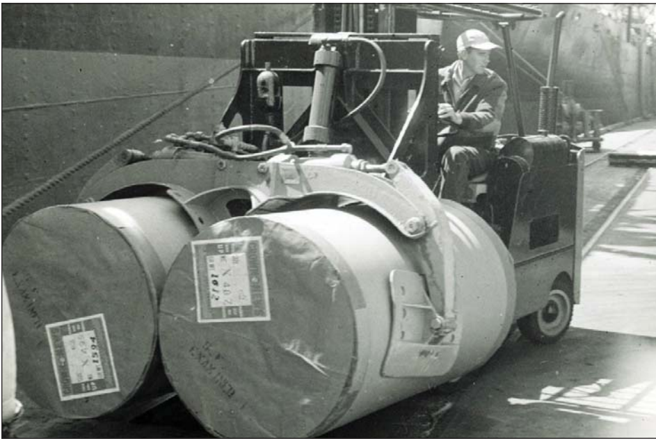
With the introduction of clamp bridles and the clamp lift jitneys in the hold, discharge of newsprint became faster, easier ... and safer for the longshoremen.
