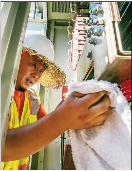
Teng Vang makes sure the substation is immaculate.
