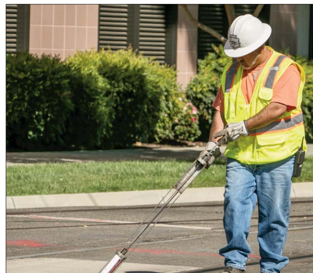
Victor Media greases a rail track.
