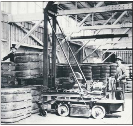
This "grandpappy of the modern forklift" at the Port of Seattle shows cargo handling and storage methods in the 1920s.
