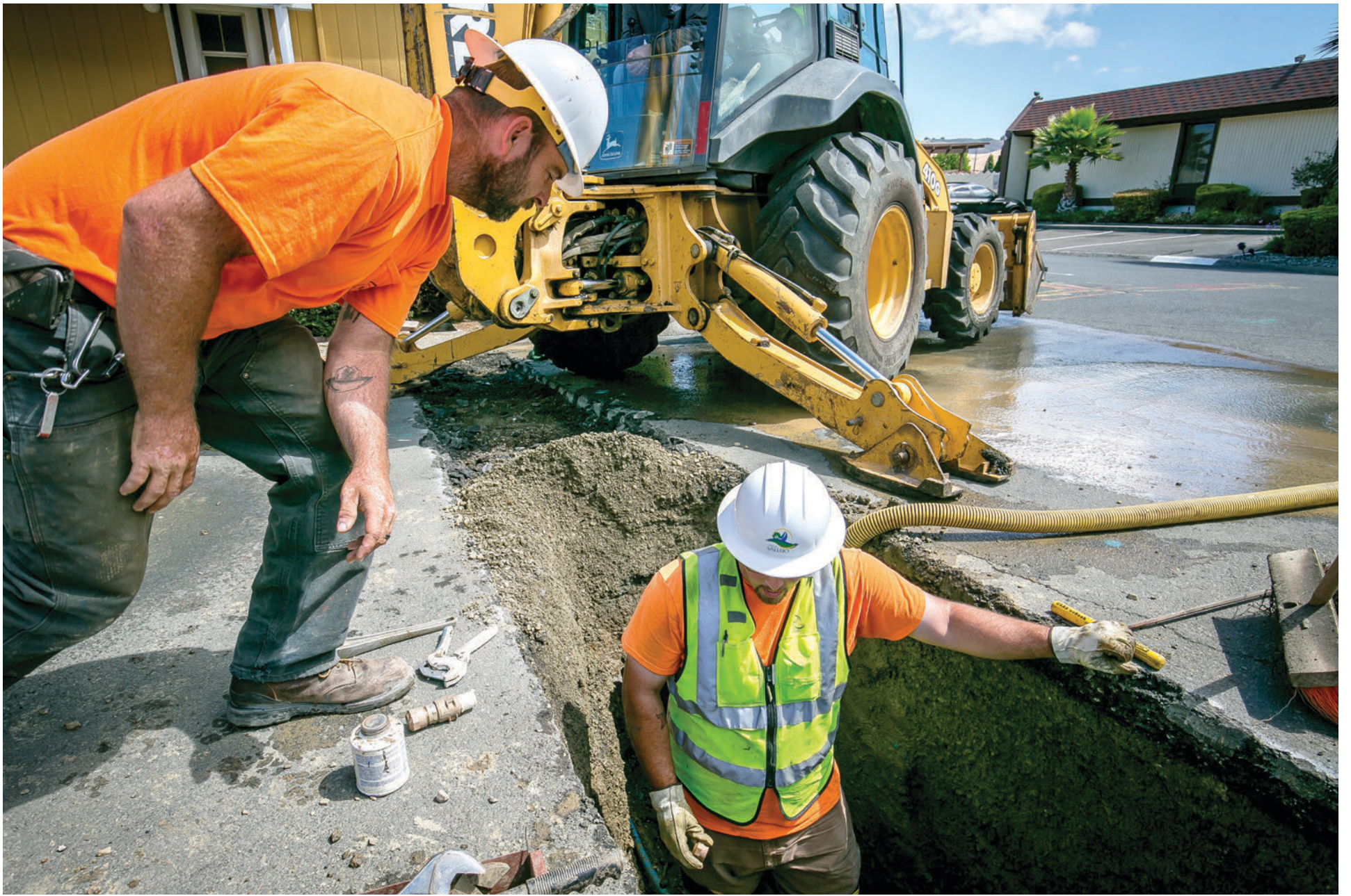
IBEW 1245 members James Grandrath, left, and Blake Peppers fix a water leak for the City of Vallejo Public Works Water Division.
