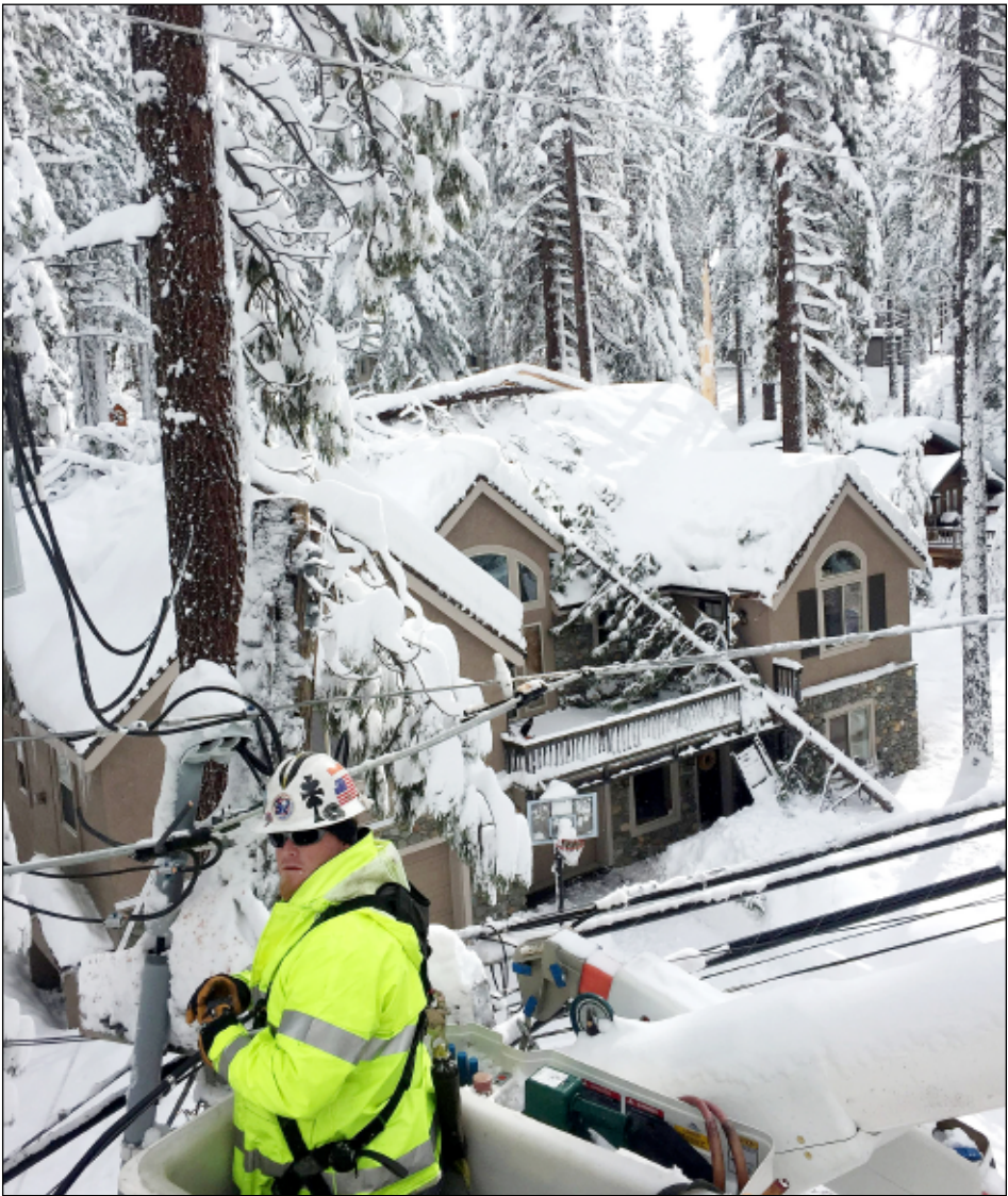
NV Energy Lineman Jeremy Parks making repairs on lines that were brought down by trees weighed down with snow. Photo by Samson Wilson
