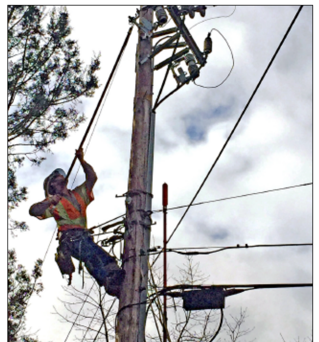
Healdsburg Lineman Brent Sullivan energizing a single phase tap line
