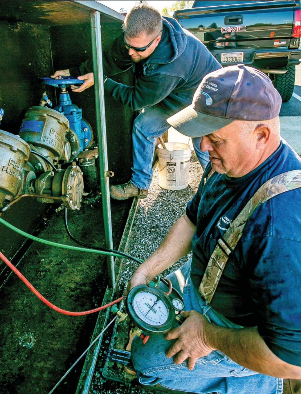
IBEW member Erick Ruste, bottom, and Curt Bloom check a back flow valve
