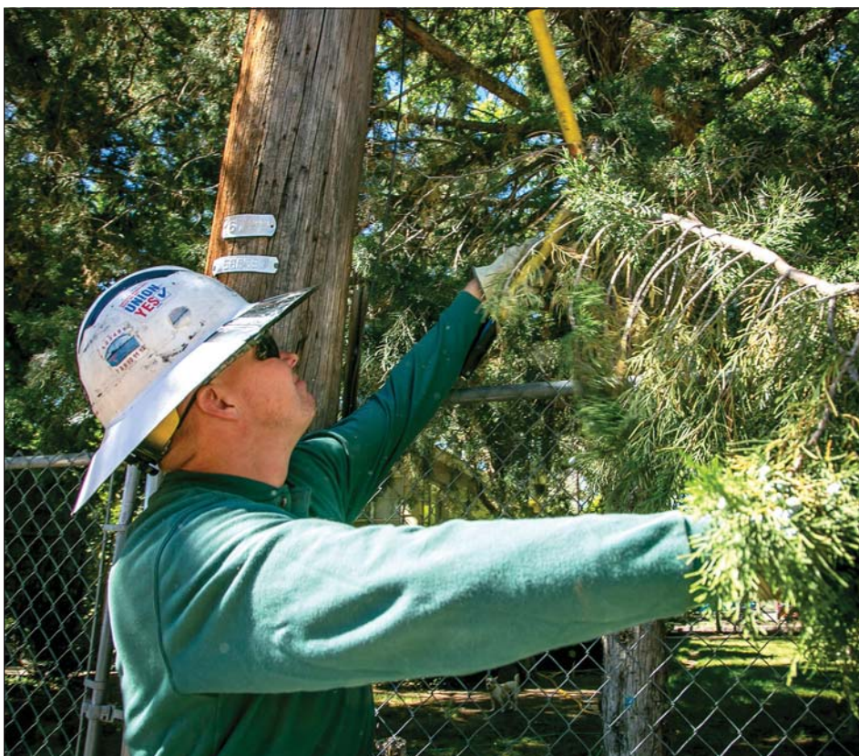
Lineman Erik Hall, whose home local is IBEW 111 in Denver, clears away the branches cut by Frank Ortega
