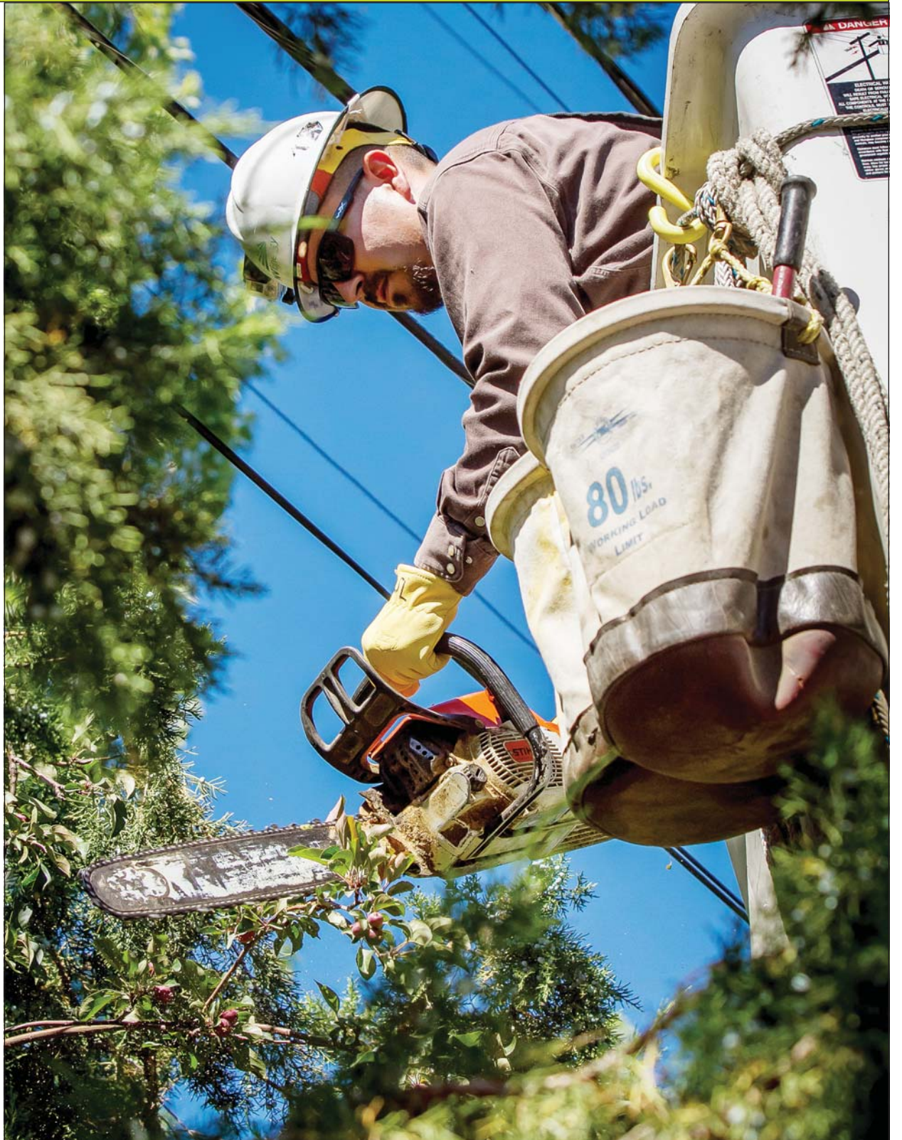
Apprentice Frank Ortega clears the way for the new conductor
