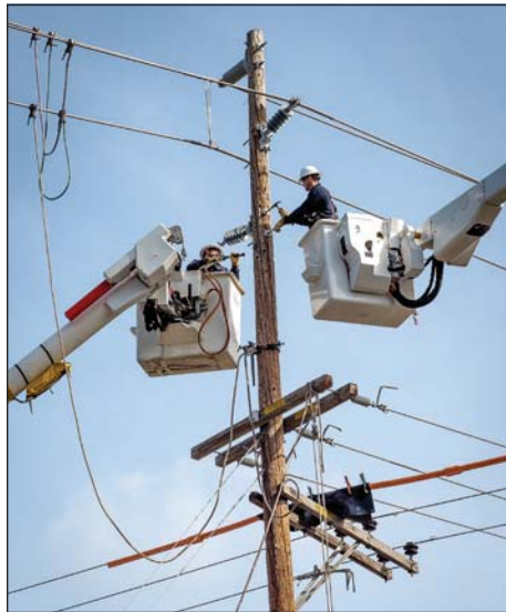
IBEW members Matt Contreras, (left), and Jesse Murrill work on a 60KV reconductor project
