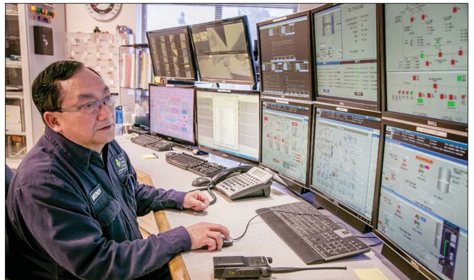
IBEW member Minh Phung works in the control room at the power plant
