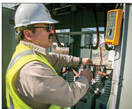
IBEW member Chris Guerrero checks capacitors at a Silicon Valley Power substation
