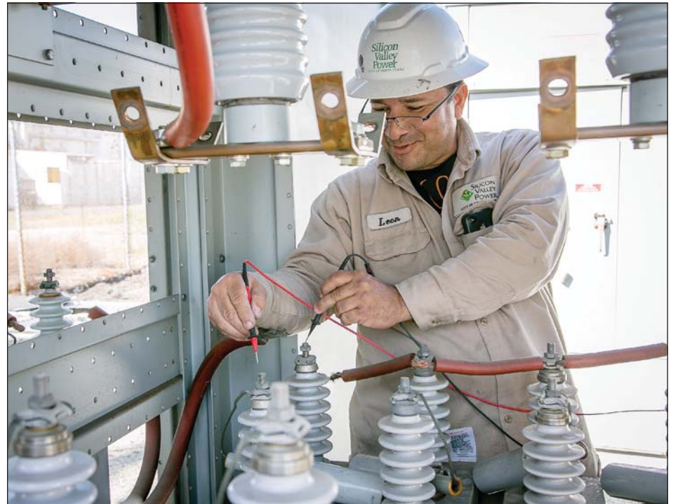
IBEW member Leon Alcantar checks capacitors at a Silicon Valley Power substation
