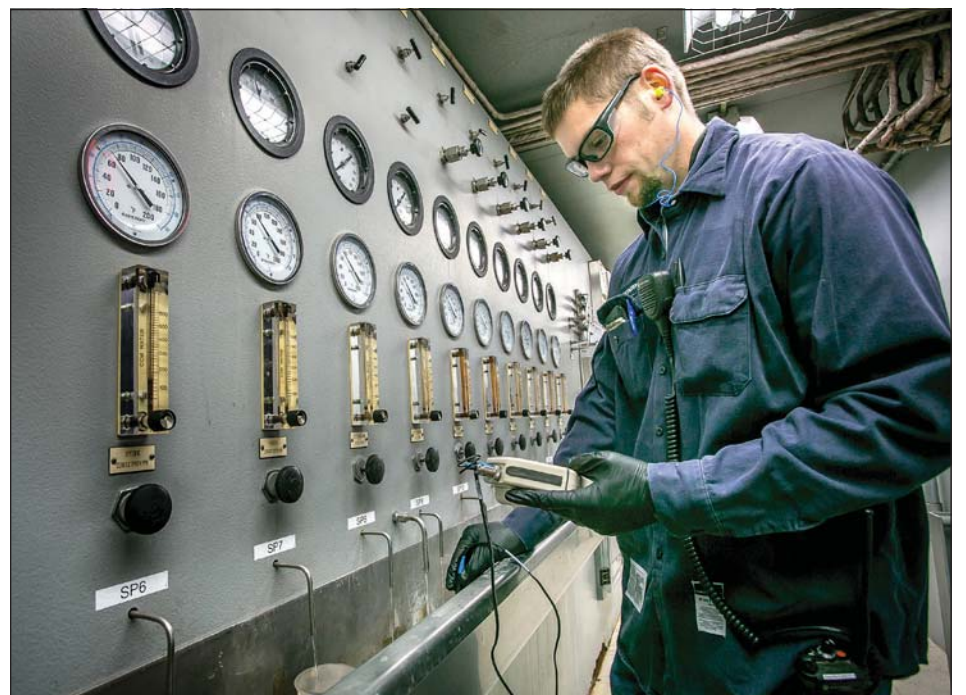
IBEW member Anthony Harnish checks the pH of the water at the gas powered generation plant for Silicon Valley Power
