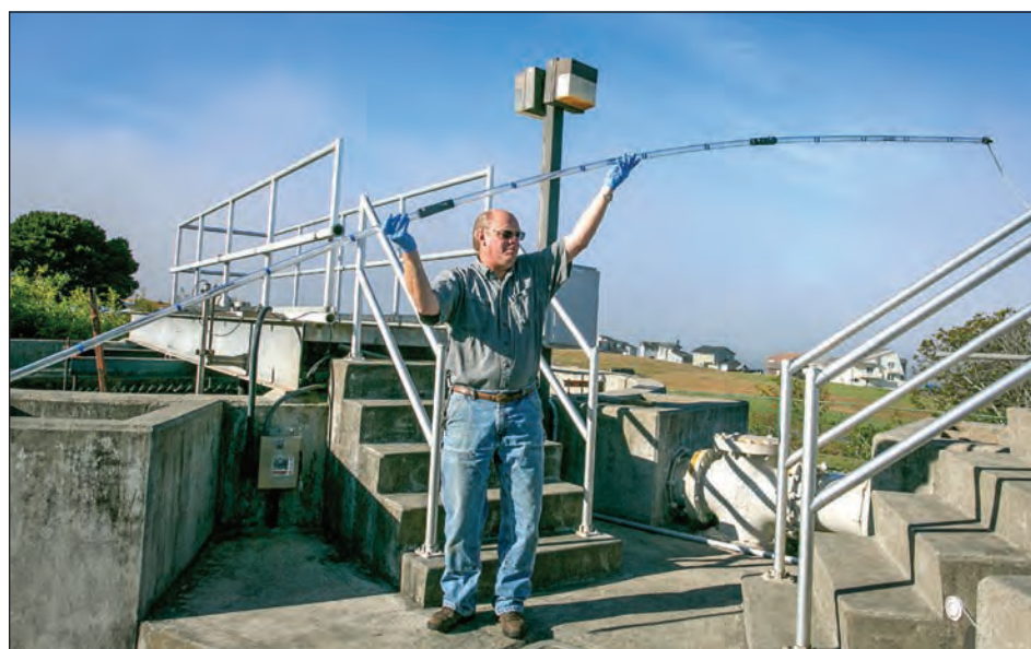
The water treatment plant services 27 miles of sewer lines through difficult terrain.
