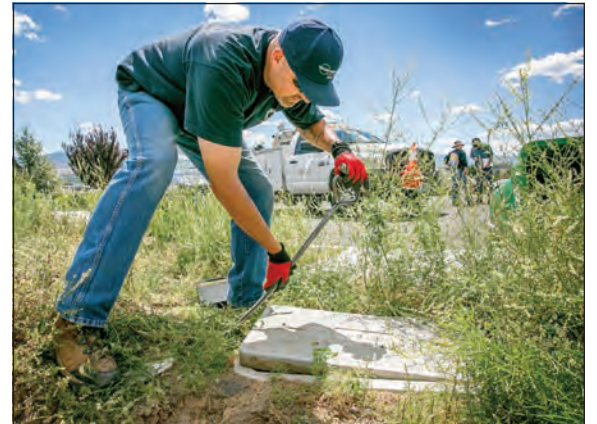
Service Tech Justin Greenland turns on water service at a residence in Reno.
