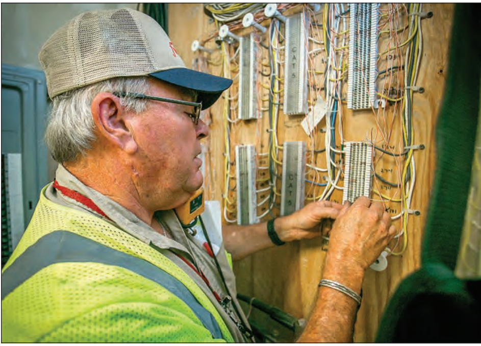
Sales & Service Technician David Mason
