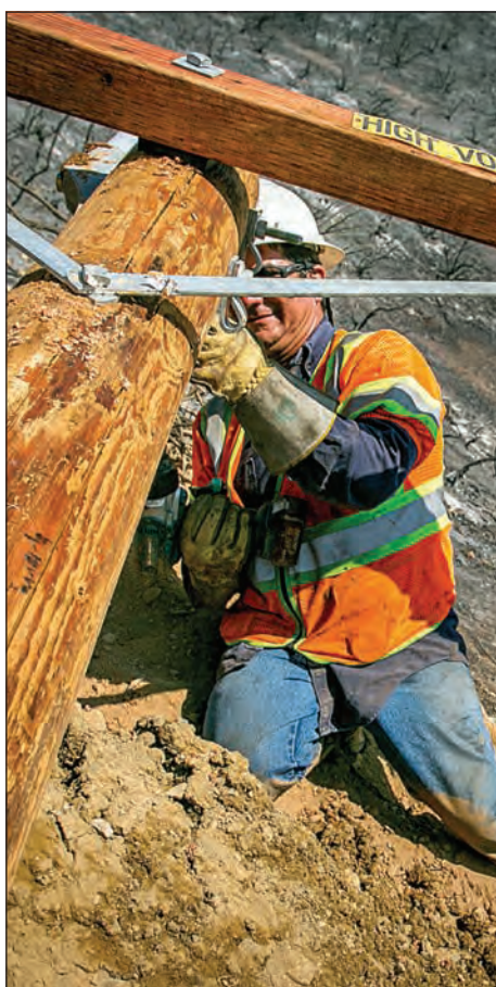
Hollis Hadley (left) and Don Lee (right) work on the new cross arms.
