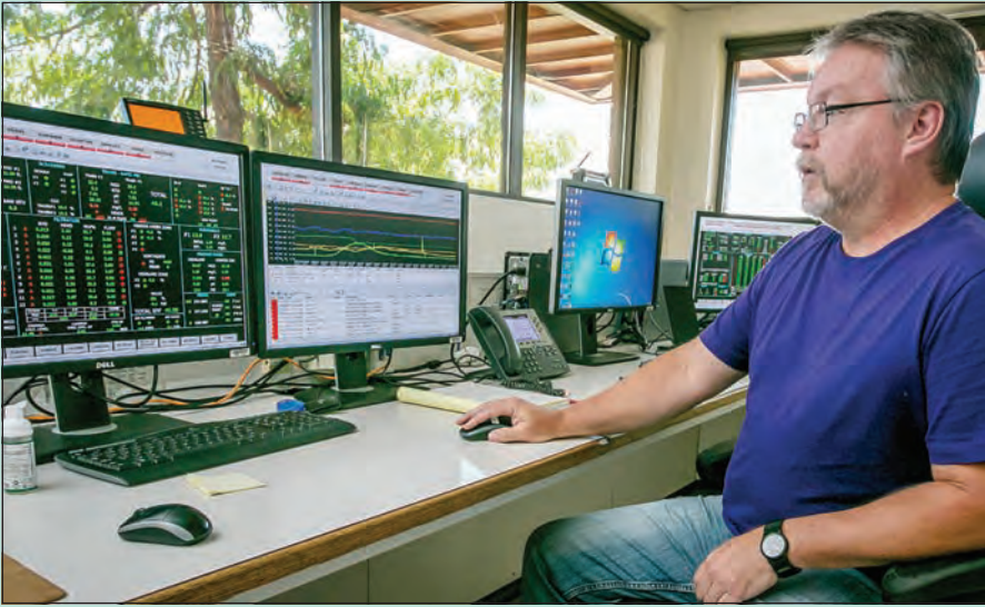
Ted Saxe, water treatment foreman, monitors treatment processes from the control room.
