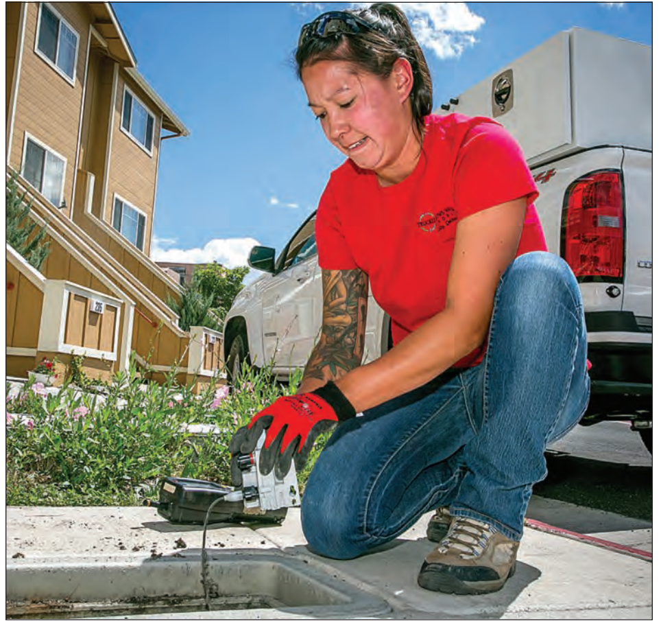
Service Utility Worker Amanda Filut checks on a transmitter at a residence.
