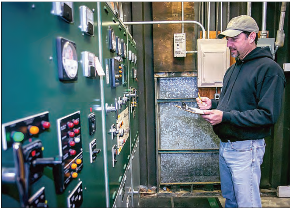
Electric Utility Superintendent Todd Nuse checks the backup generators.
