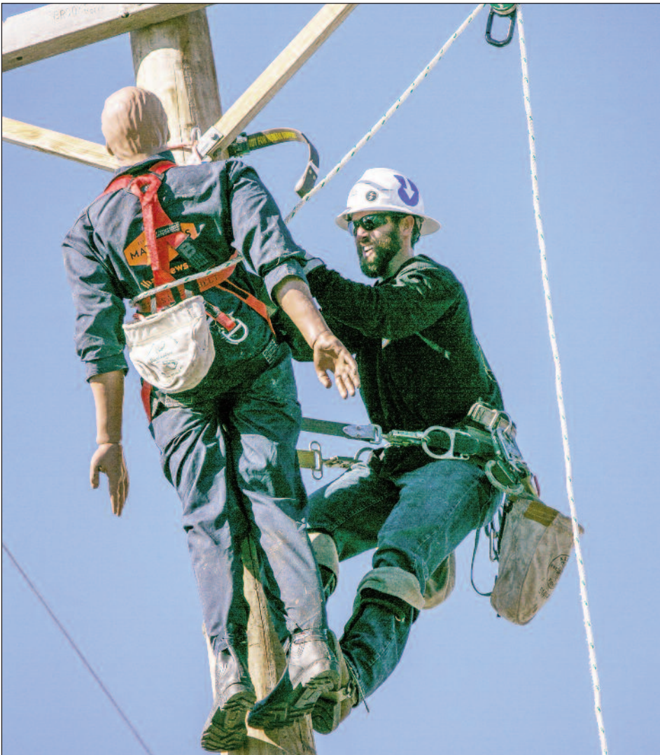
Apprentice Michael Anderson, Outside Construction
