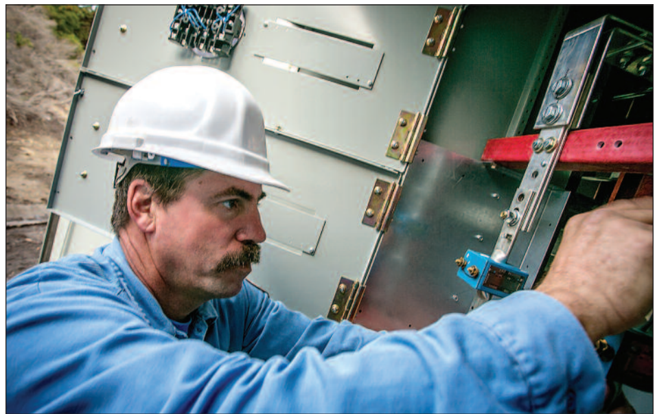
Alvin Allen, Substation Tech, installs metering equipment.
