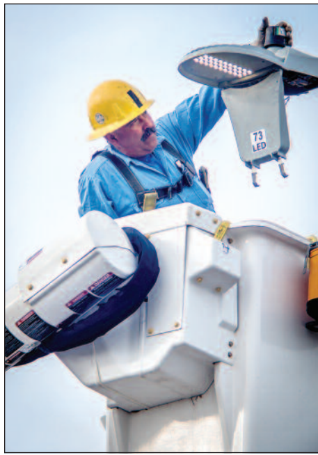
Tony Vickery, Lineman, installs a new LED light.
