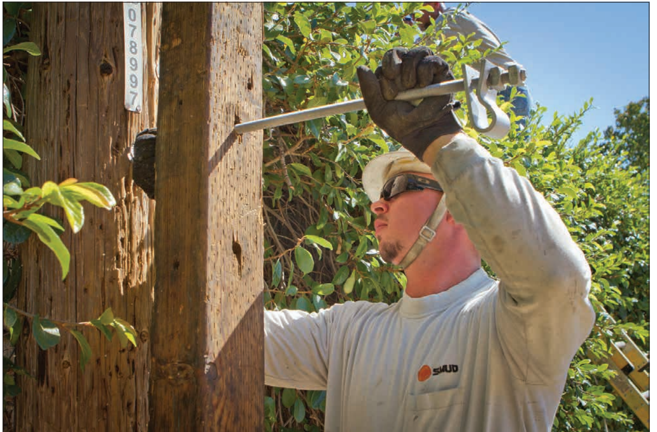
Chris Miles installs the peg leg on the pole that is to be removed.
