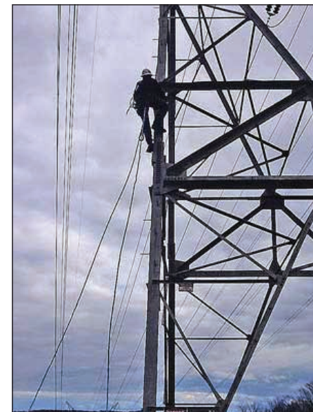
Lineman Jason Madigan ascending tower to begin job.
