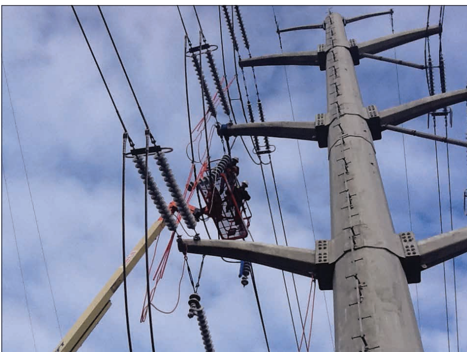
Terry Daniels led crew replacing transmission bells in New Castle. Linemen Eric Willis and Joe Bryant in man basket.
