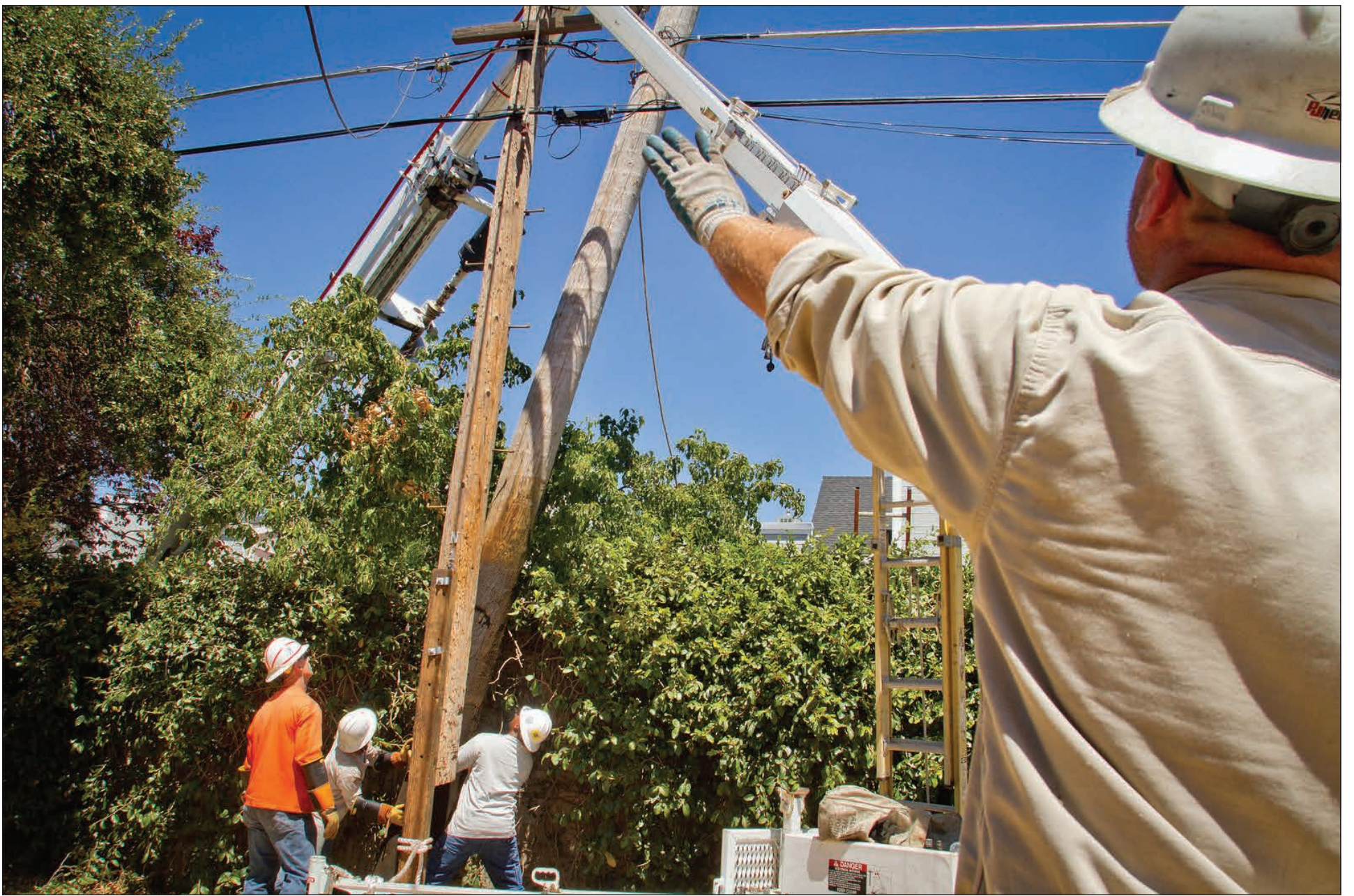
The crew maneuvers the new pole into place alongside the old one.
