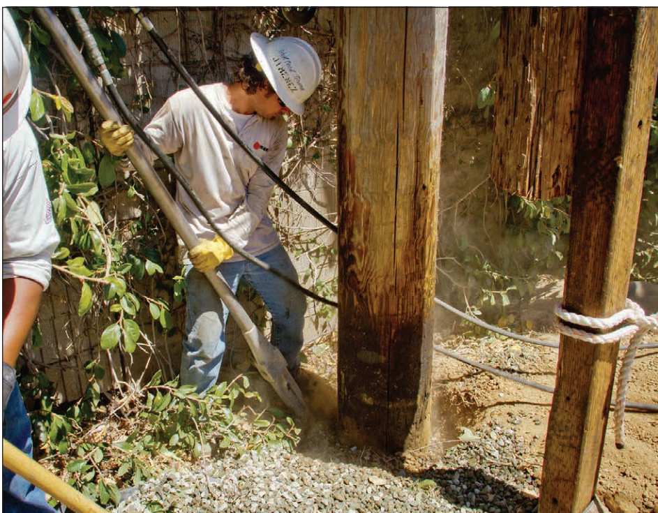
Louis Jimenez uses hydraulic tamp to tamp gravel around the new pole.
