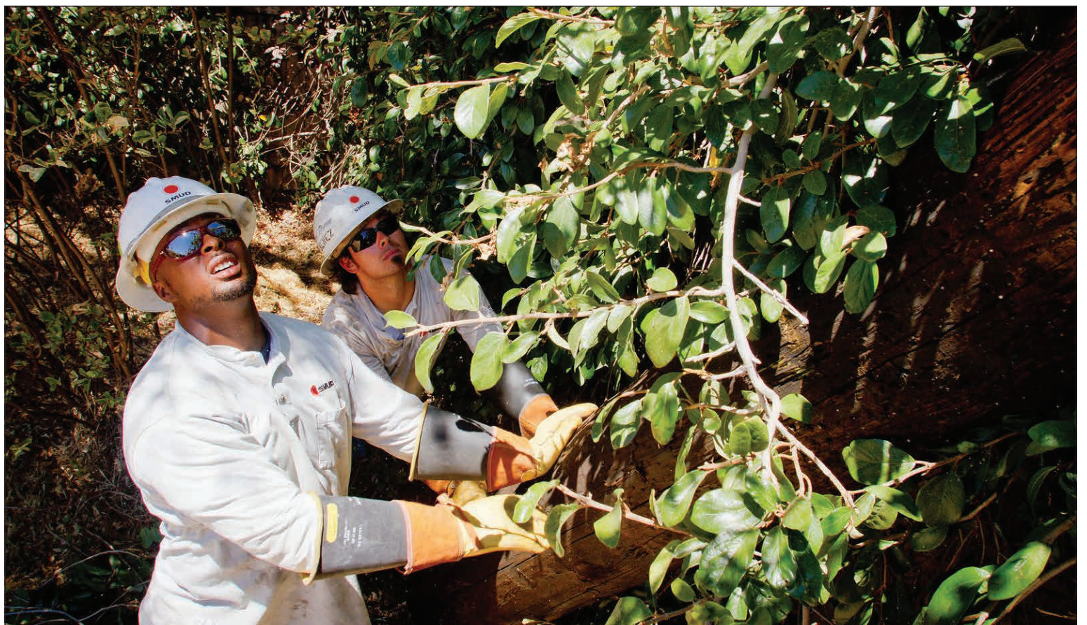
Wesley Simmons, left, and Louis Jimenez control the butt of the new pole as it is positioned.
