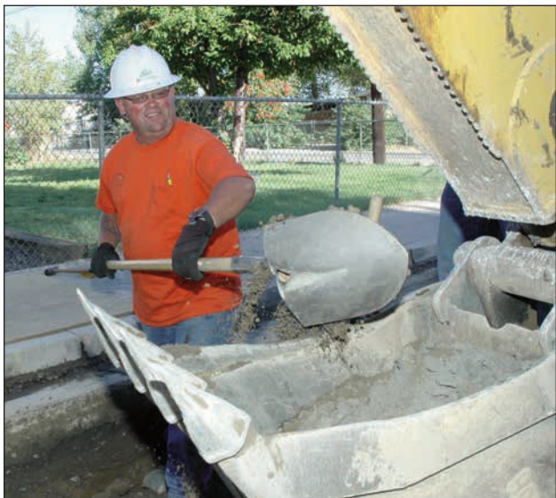
Cliff Pinkham, Apprentice Fitter, removes spoil.
