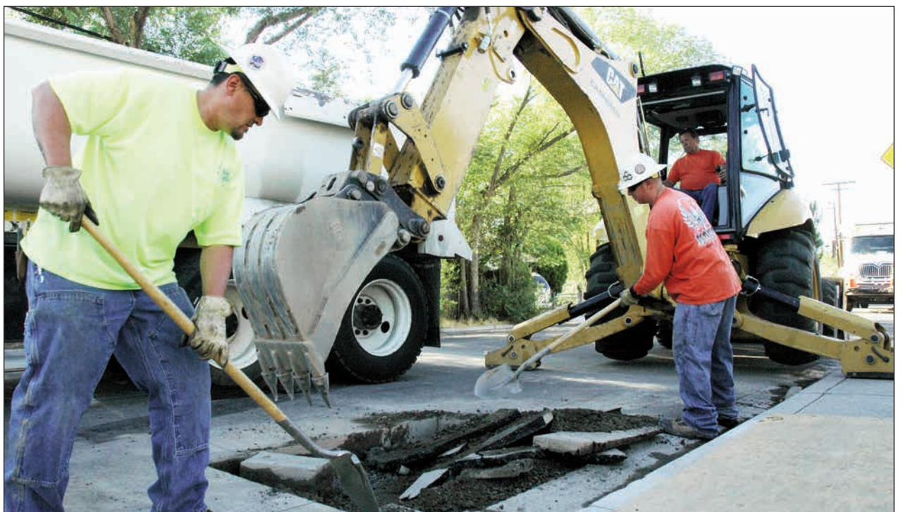
Beginning to dig is Robert Belles (in backhoe), assisted by Robert Fintland and Marty Krumle.
