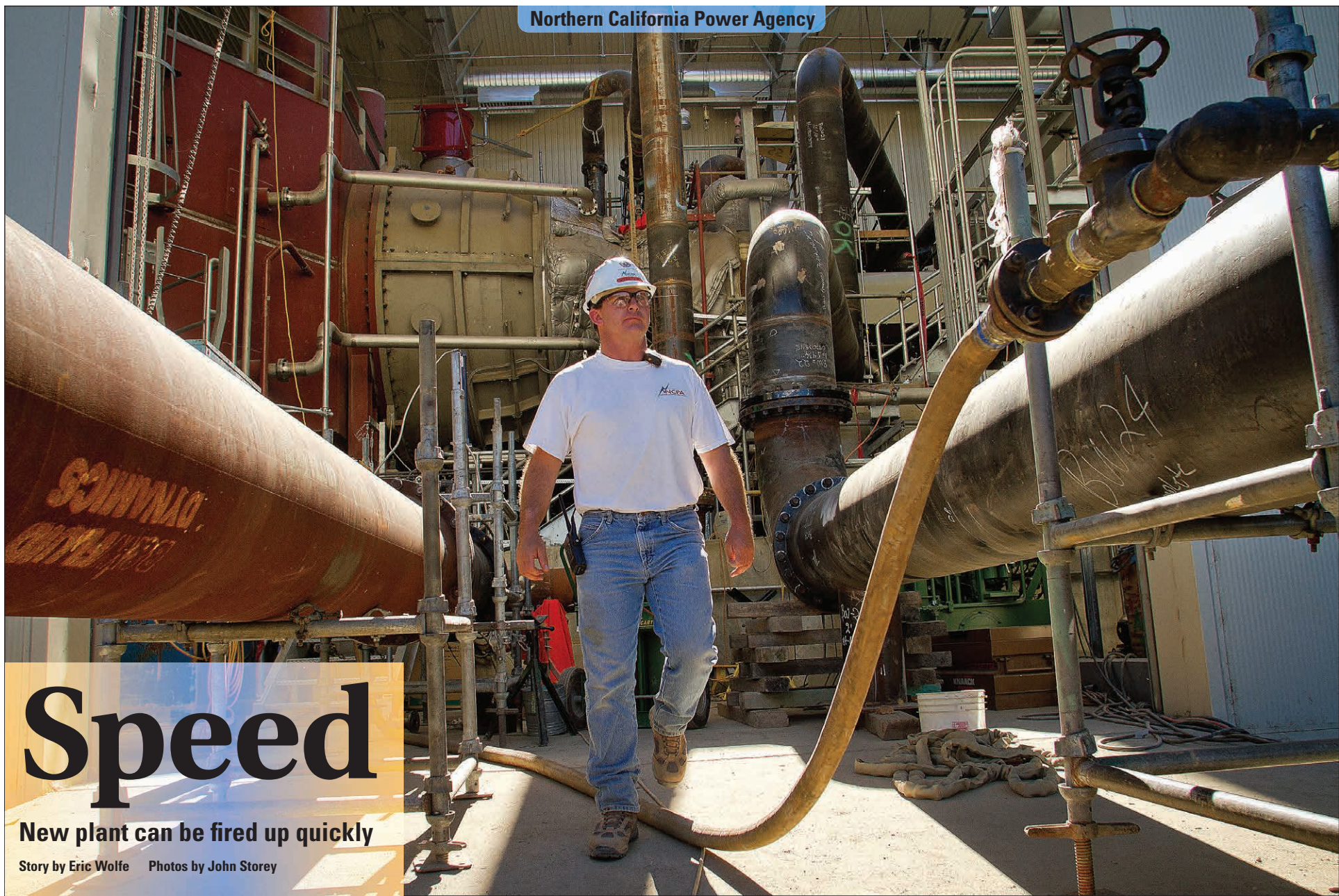
John Quitter walking outside the Steam Turbine building during steam blows with temporary piping installed.
