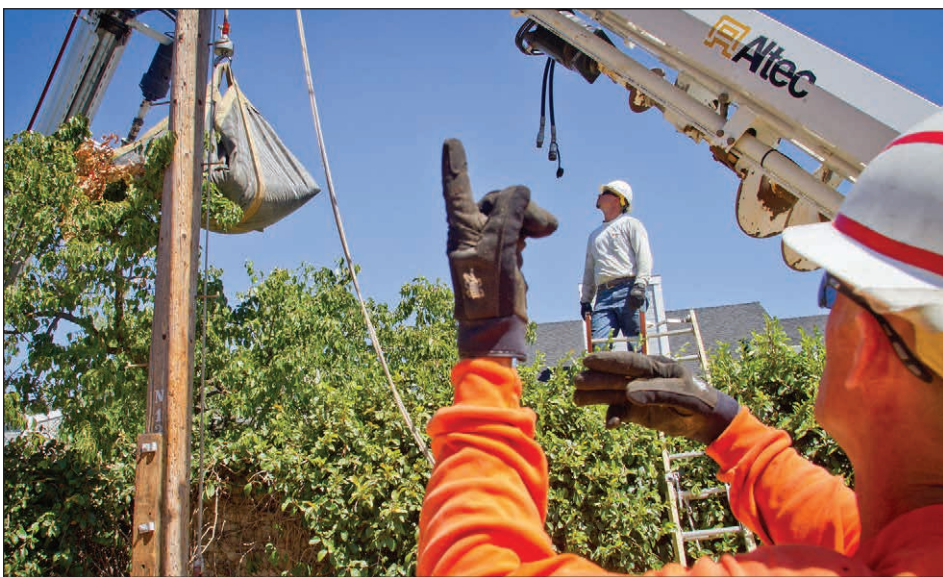
The crew maneuvers the new pole into place alongside the old one.
