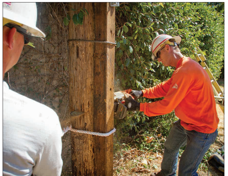
Jeremy Mashall cuts the pole after it has been attached to the peg leg.
