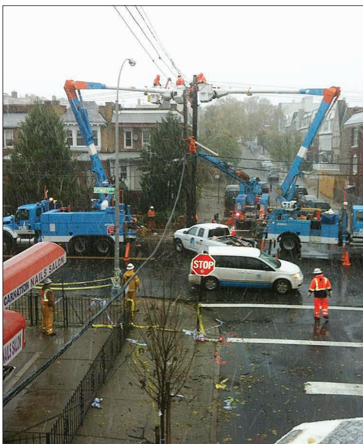
IBEW members from PG&E were part of a massive restoration effort in November in the wake of Hurricane Sandy.
