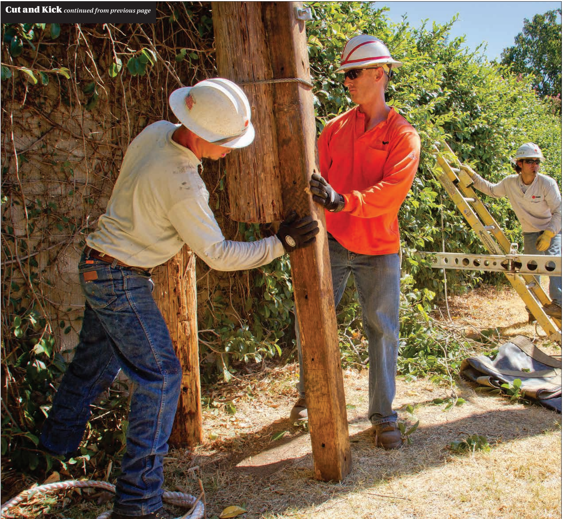
Moving the top of the old pole to make room for removing the butt.
