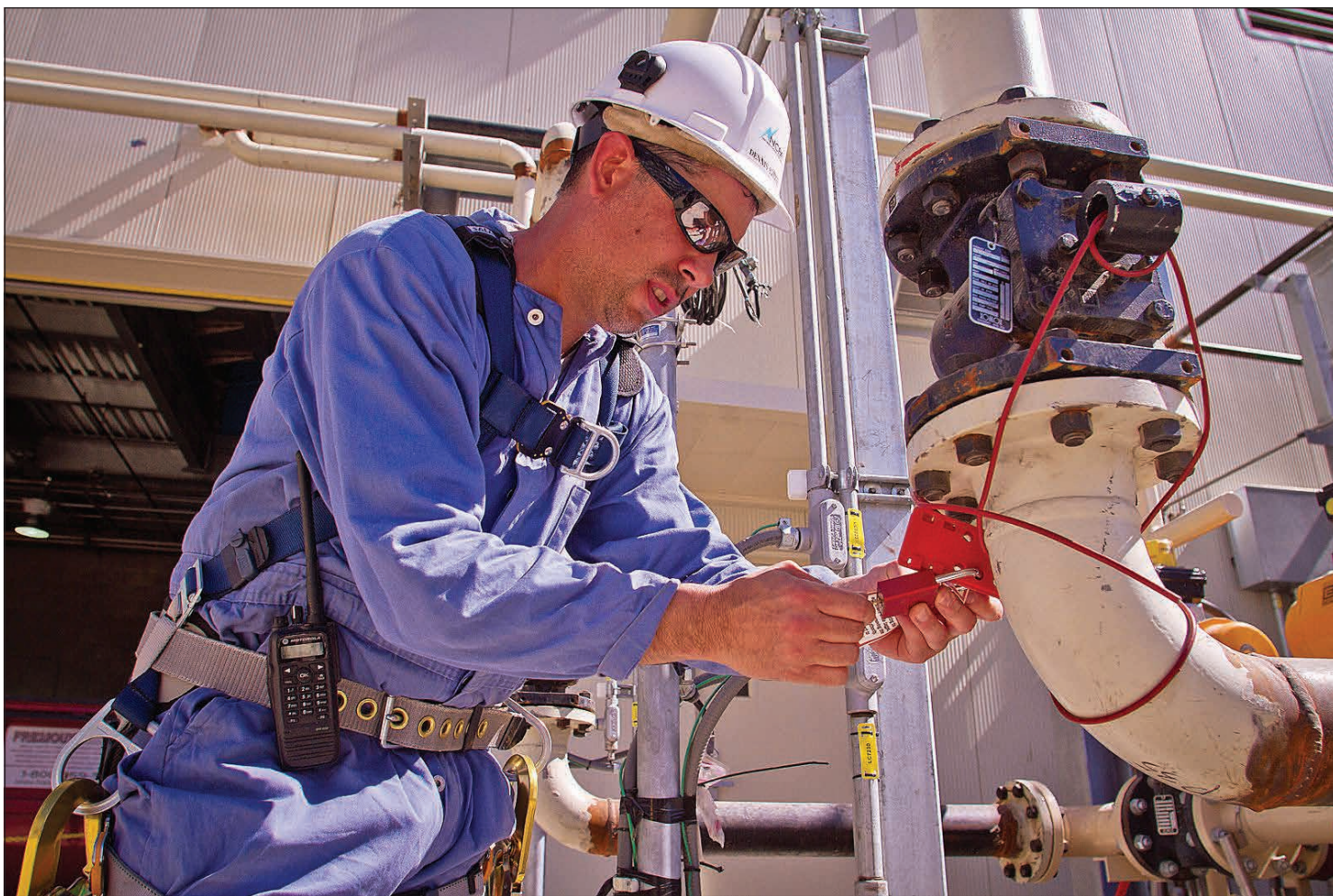
Dennis Stimac (Combustion Turbine Specialist) locking a valve shut on a filter press forwarding pump.
