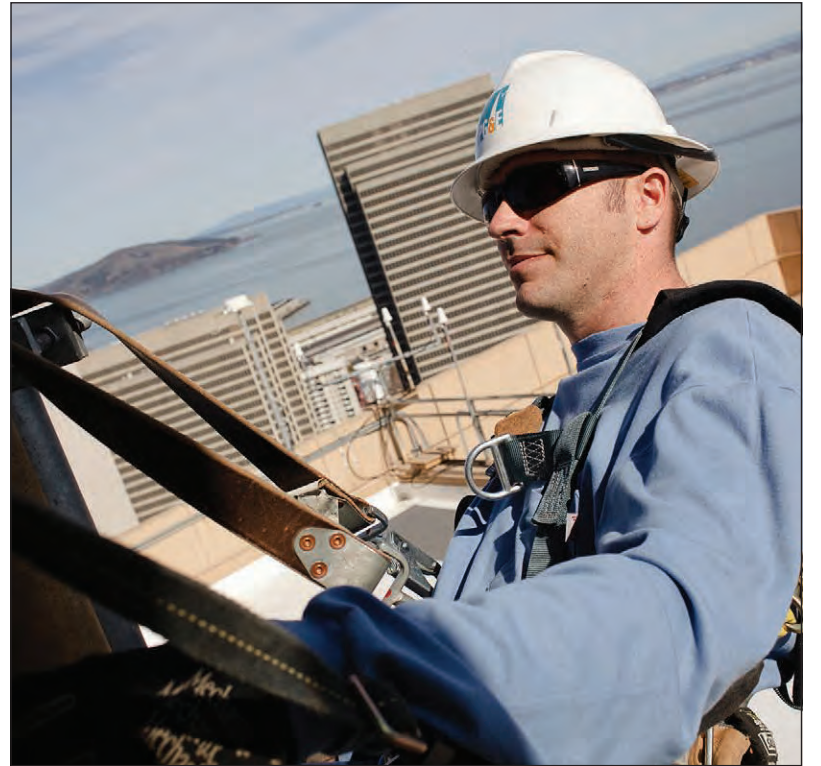
Anthony Jones works on the antenna installation.
