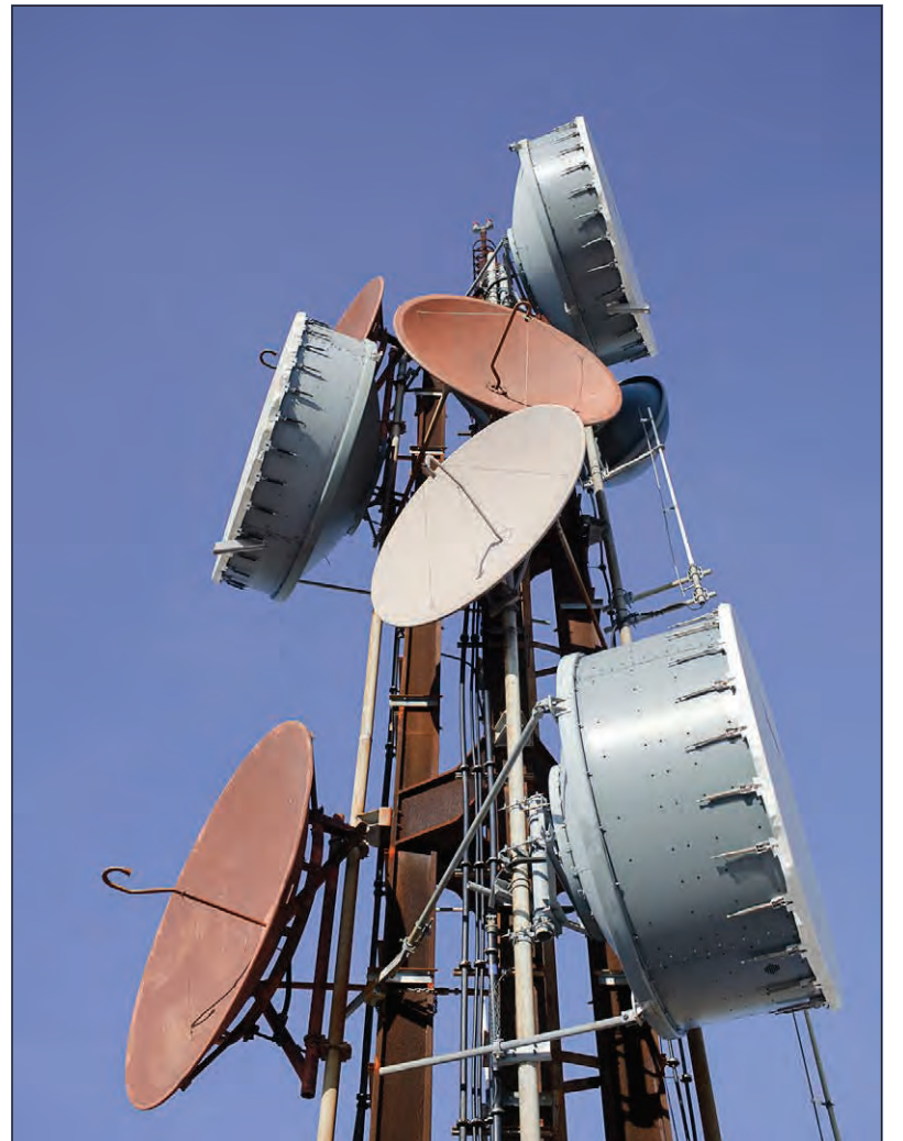
Communications equipment on top of 77 Beale permits PG&E to gather information from around its system.
