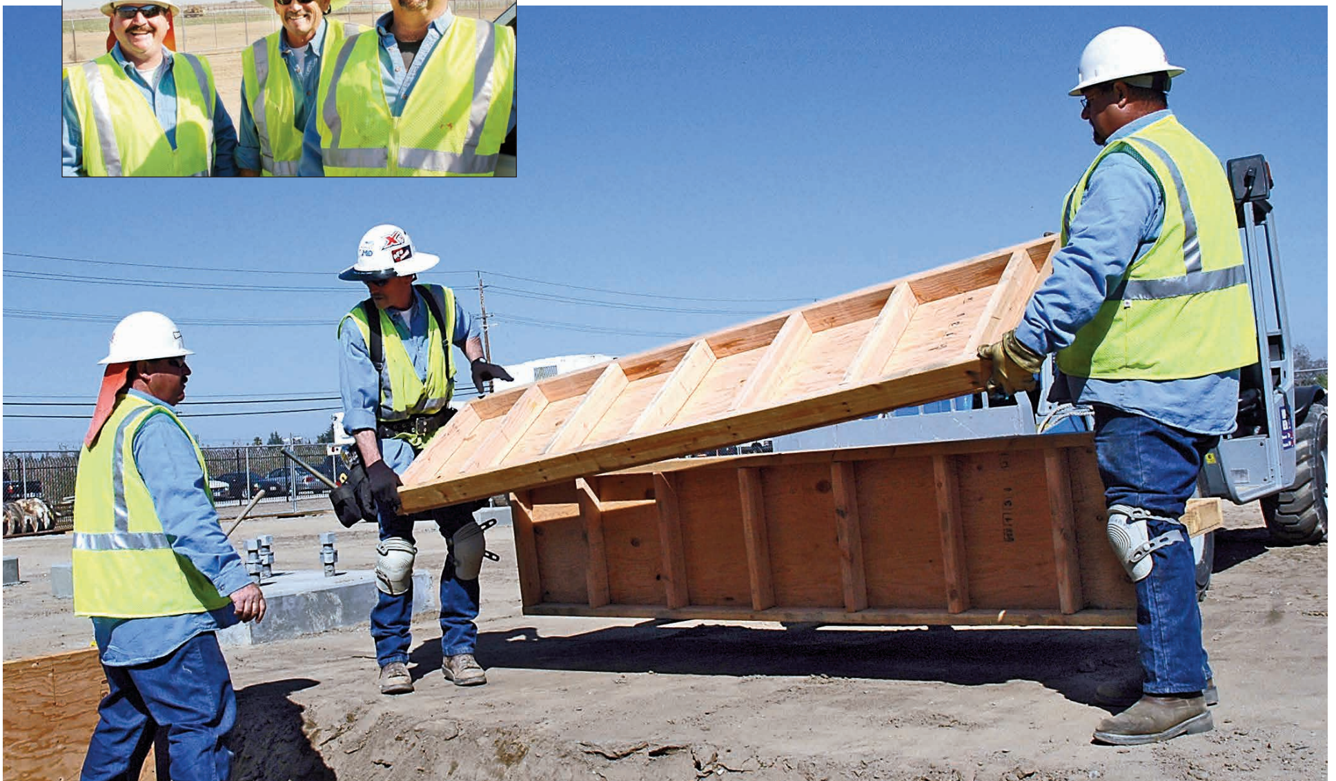
Building forms for the foundation are, from left, Ty Thatcher, Tony Moore and David Tremayne.
