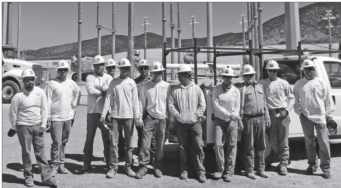
Local 1245 members working for Wilson Construction are building the Robinson Substation on 90 acres about an hour's drive outside Ely, NV. Started in 2011, the sub is scheduled to be completed in late 2012. It will not become operational until 2014, due to delays in the SWIP Transmission Line it will connect to. General Foreman on the job is 45-year IBEW member Larry Paul. Photo by Ron Cochran
