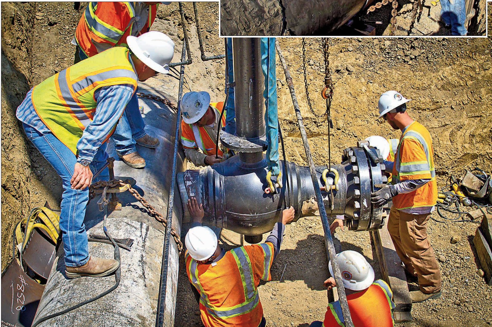
(Below) Tapping into the 32-inch line.
