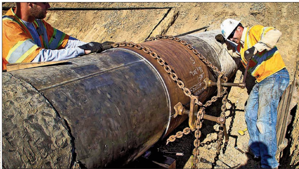
(Right) Pat Ming, right, tightens the sleeve with a chain-style sleeve jack. At left is Donovan Odle.
