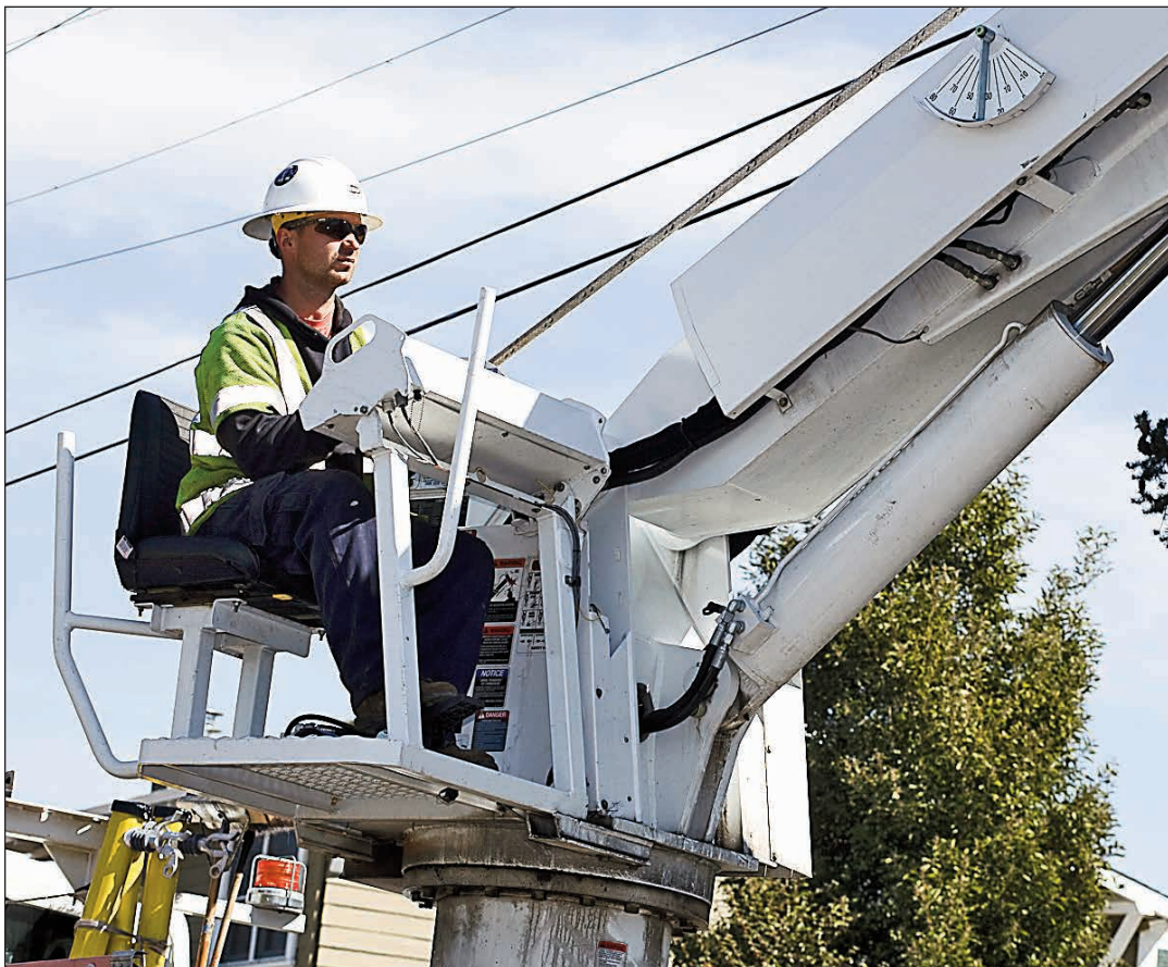
Lineman Vlad Derevnyuk operates the boom.
