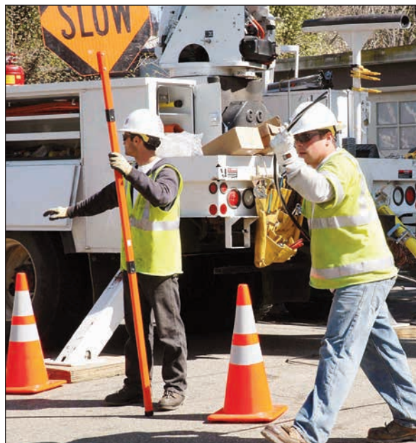
Groundman Cornell Fechete control traffic while Jeremias Arevalo runs a service to a house.
