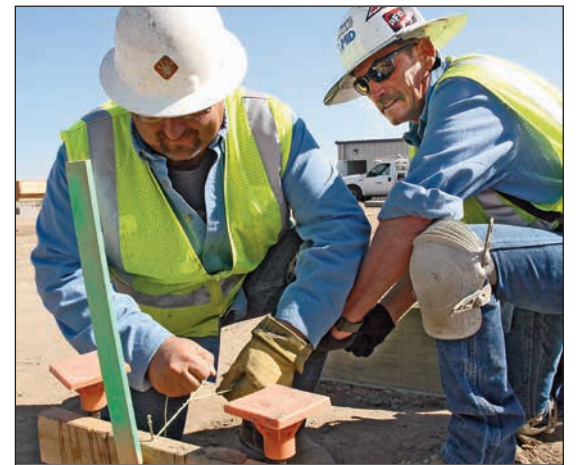
David Tremayne and Tony Moore at work building the forms for the foundation.
