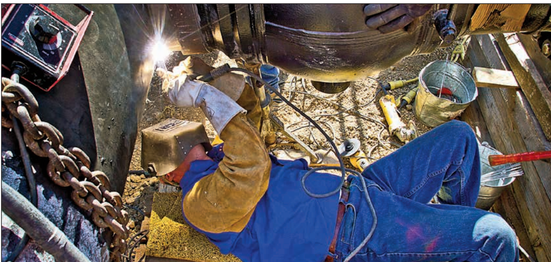
Mauro Cortes, welding.
