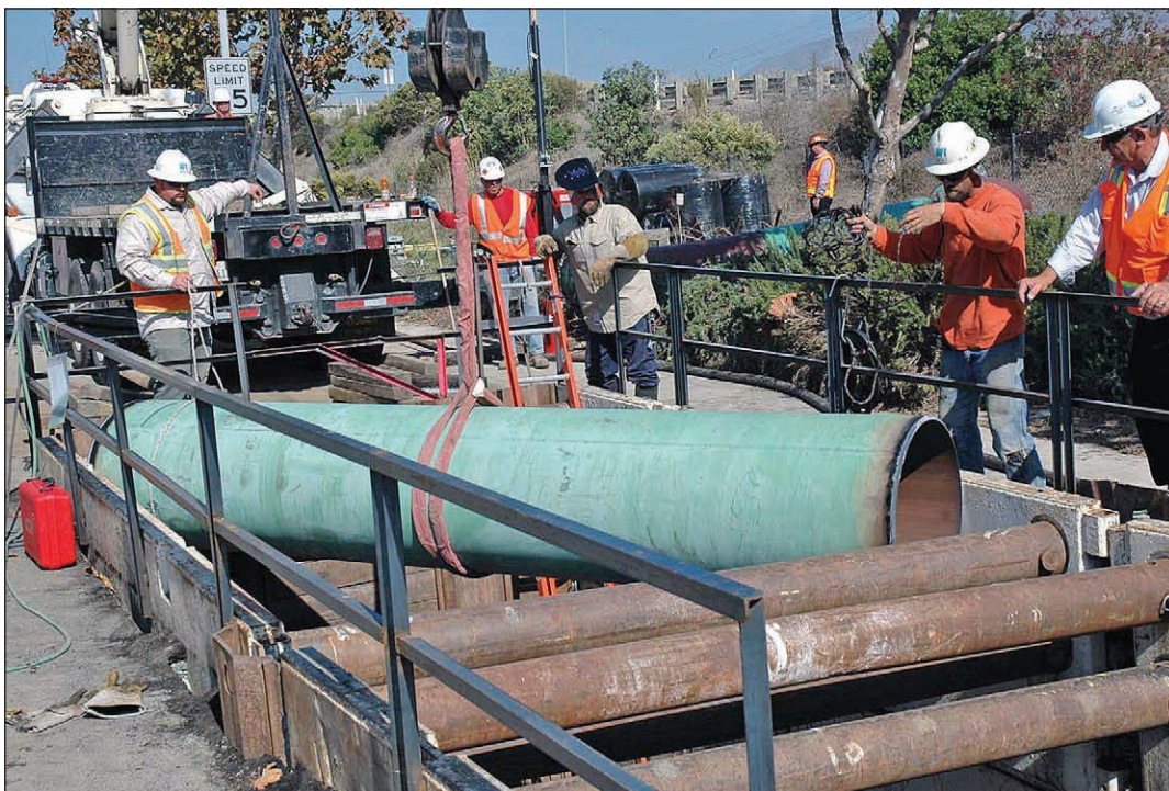
The pipe is carefully maneuvered into the narrow space through which it will be lowered into the vault.
