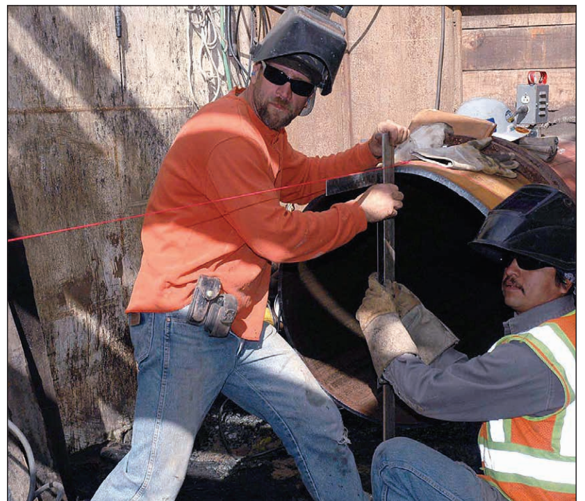
Making sure the ends of the pipe are aligned.
