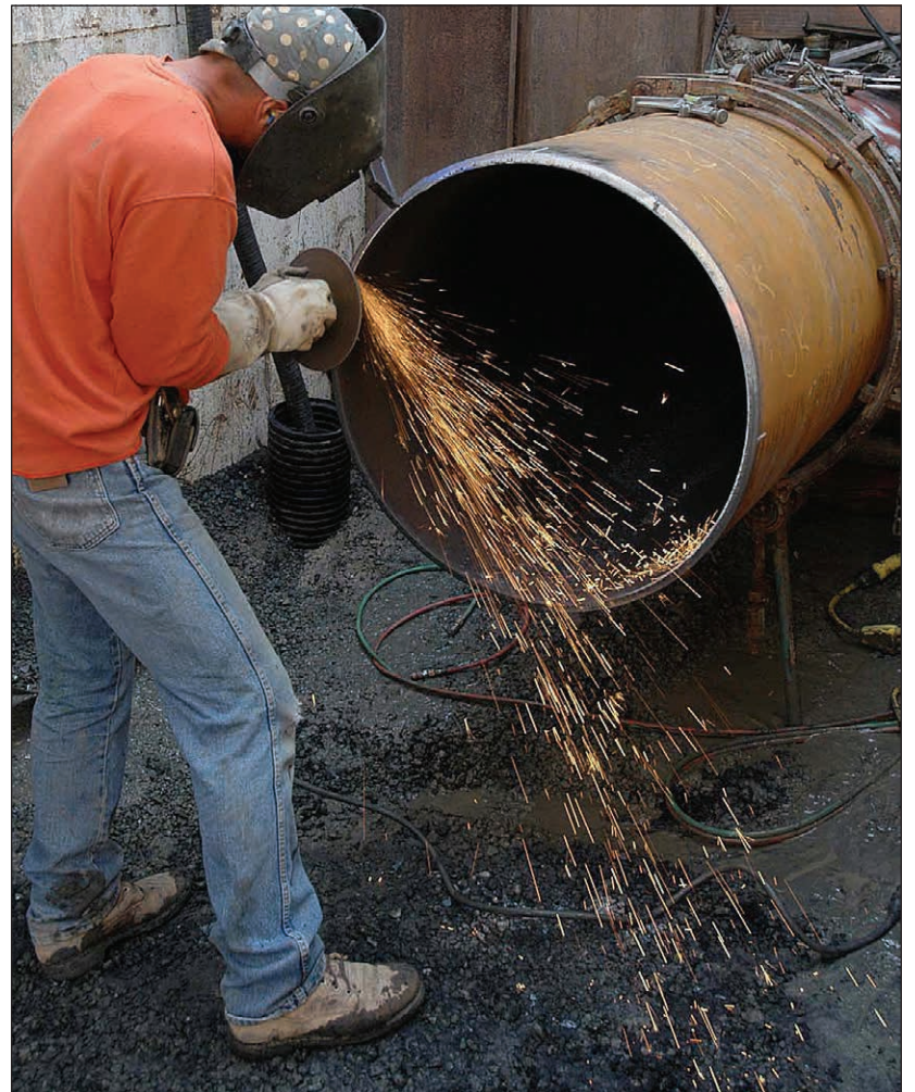
Prepping the pipe ends to weld.
