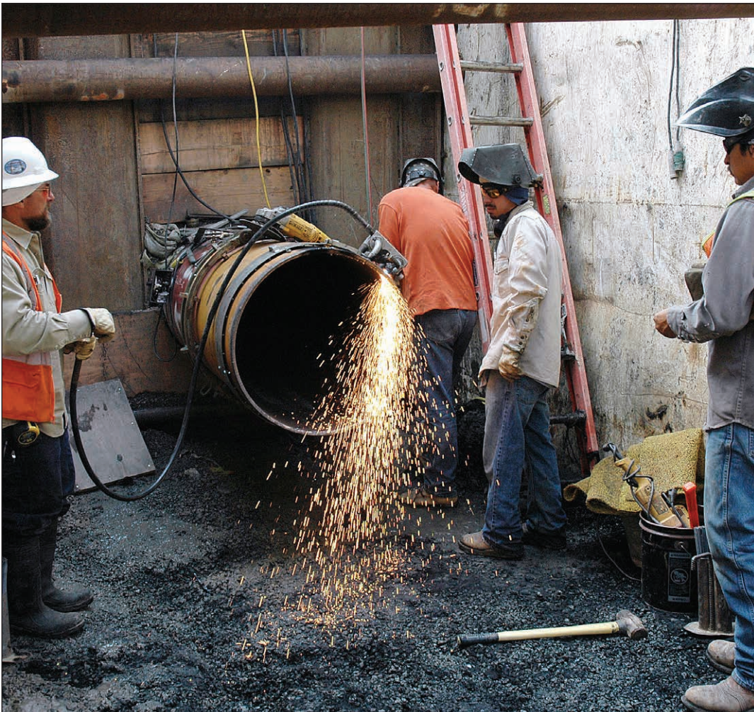
Sparks fly as the pipe is beveled.
