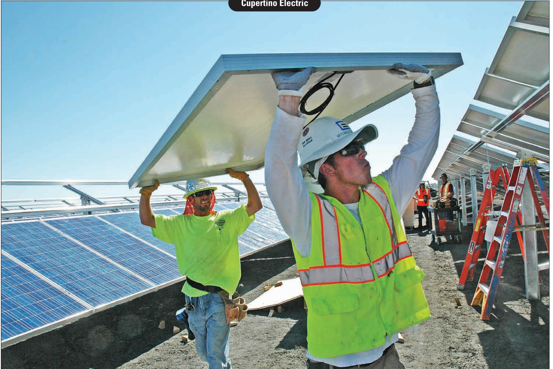
Jayson Beyer (left) and Mitchell Devenny (right) prepare to lift a panel onto the rack.
