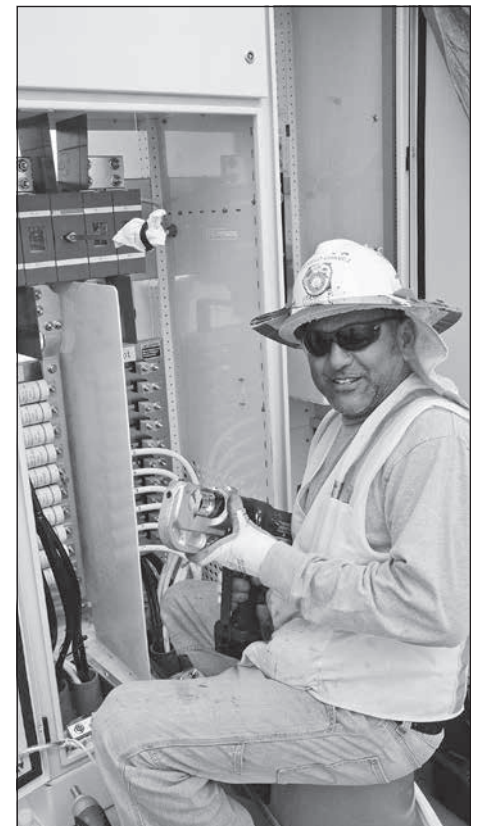
Journeyman Wireman Marcel Chavez terminating cables at an inverter.
