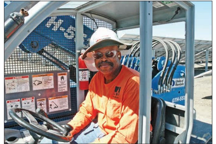
Charles Bynom, Jr. is one of seven Line Equipment men who are responsible for site logistics at the 20 MW site.
