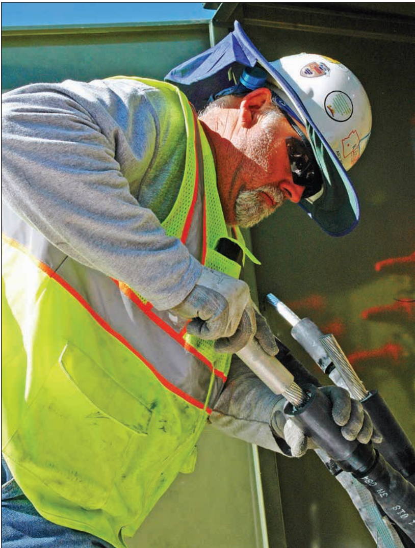
Cable Splicer Arthur Hamrick terminating a medium voltage transformer.
