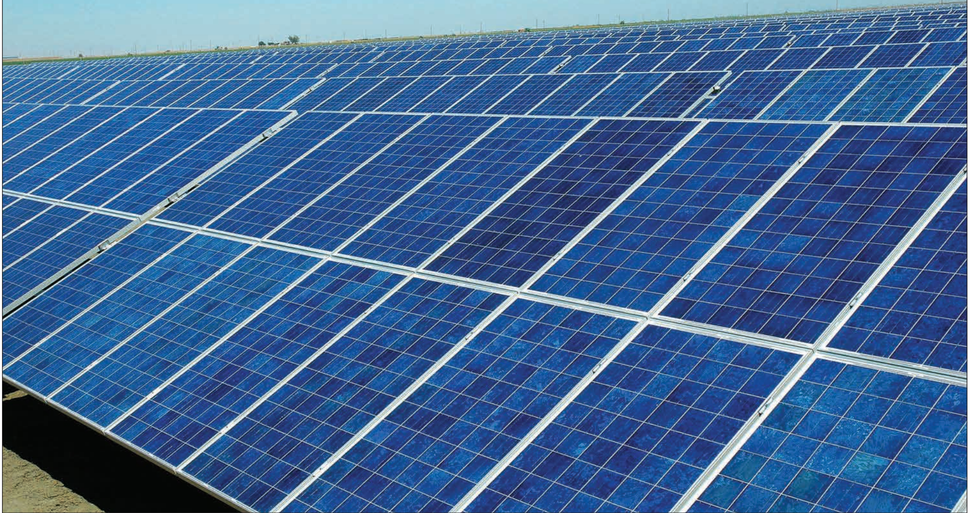
The project will use about 100,000 panels to generate 35 megawatts of electricity.
