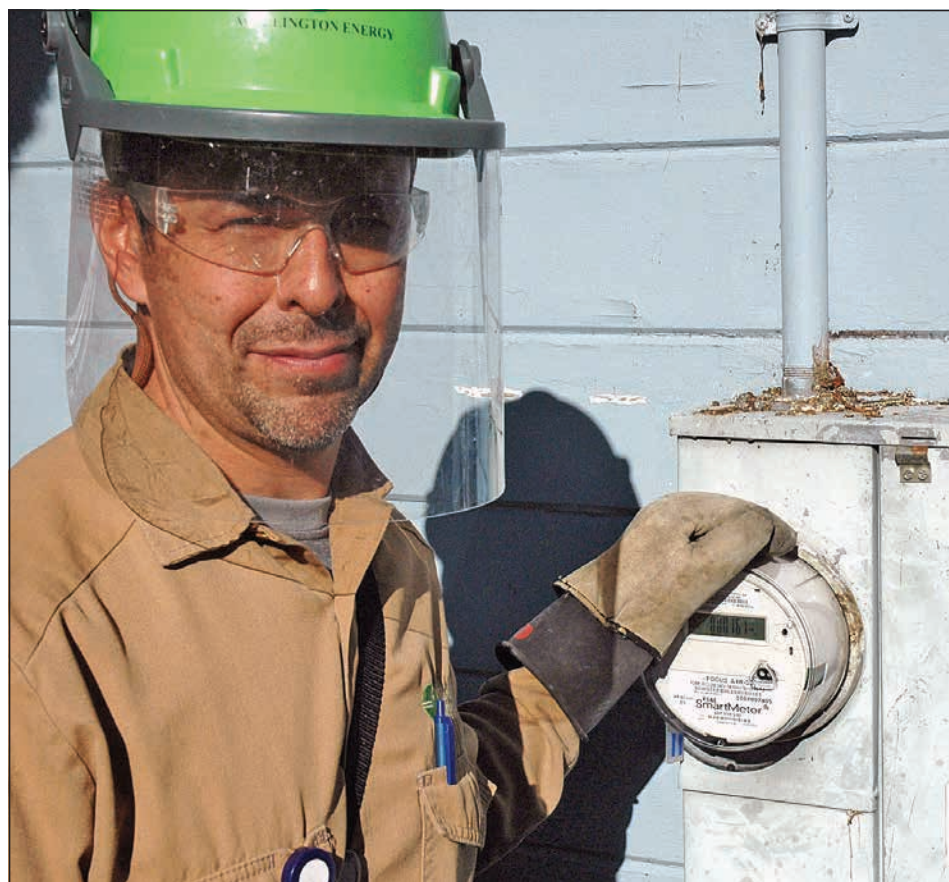
Wellington Meter Technician Orlando Miramontes removed an old PG&E electric meter and shows off the new SmartMeter he's installed in its place.
