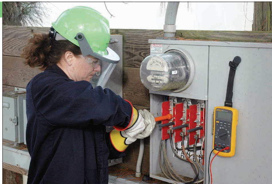
Stacy Wallace, a journeyman wireman for Wellington Energy, removes the old electric meter powering a rural residence in Sonoma County.
