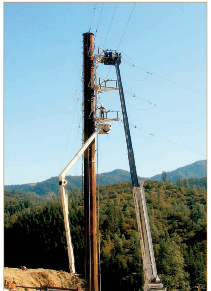
IBEW members Greg Young, Jim Deptuch and Charlie Appleton prepare to adjust 3-way 69 kv switches.
