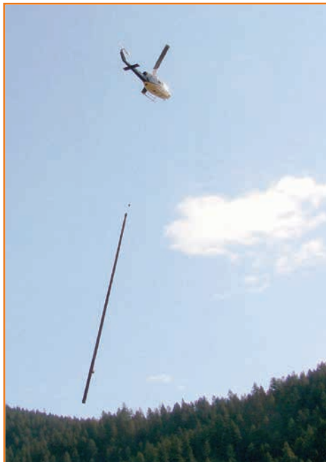
214 flying last pole to "H" structure. Pole weight is 5,600 pounds. Lift capacity is 6,000 pounds.
