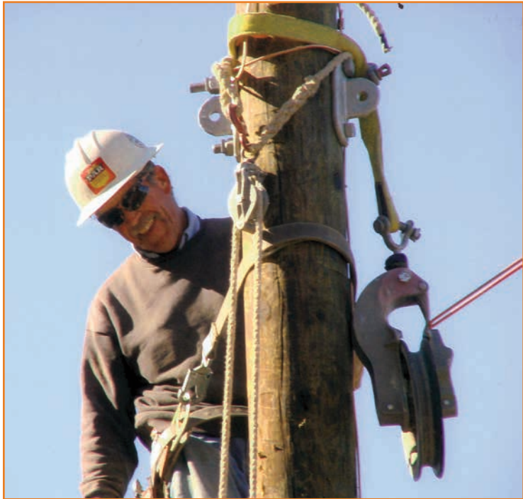
IBEW member Tim Riddle on dead-end pole.
