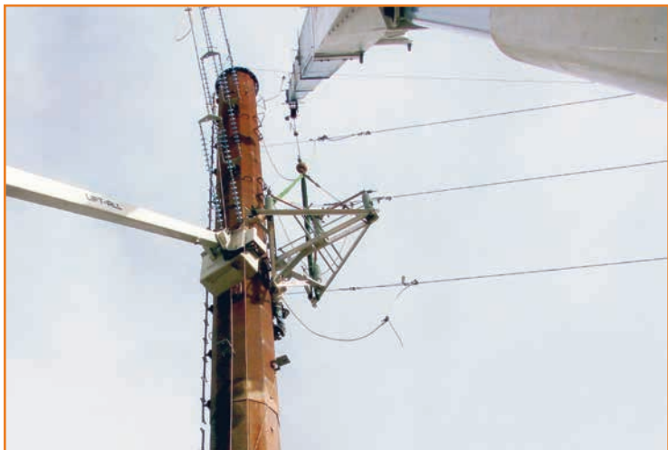
IBEW members Greg Young, Jim Deptuch and Charlie Appleton land 3-way 69 kv switch.
