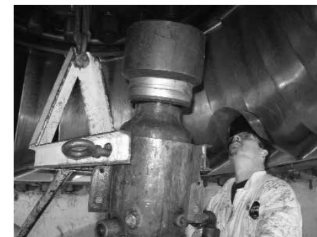
Plant Mechanic Jeff Fuller at work beneath the turbine.
