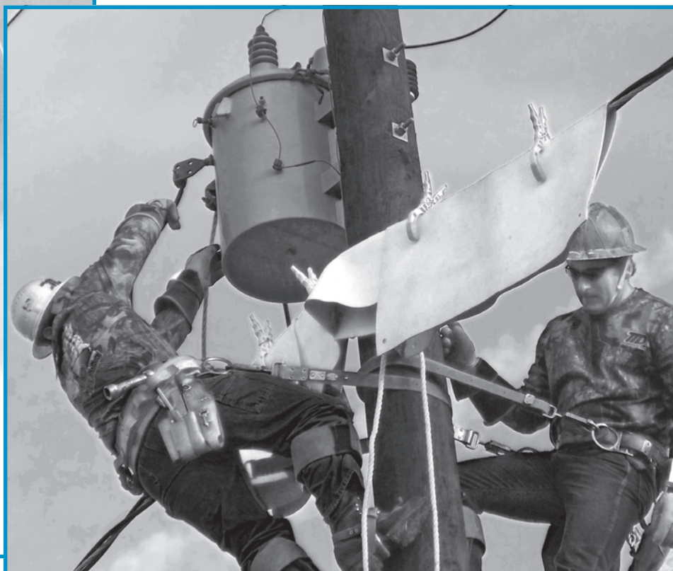
Dustin Kreiger, left, and Mark Pickens compete in the Transformer Change Out for Turlock Irrigation District, finishing third.
