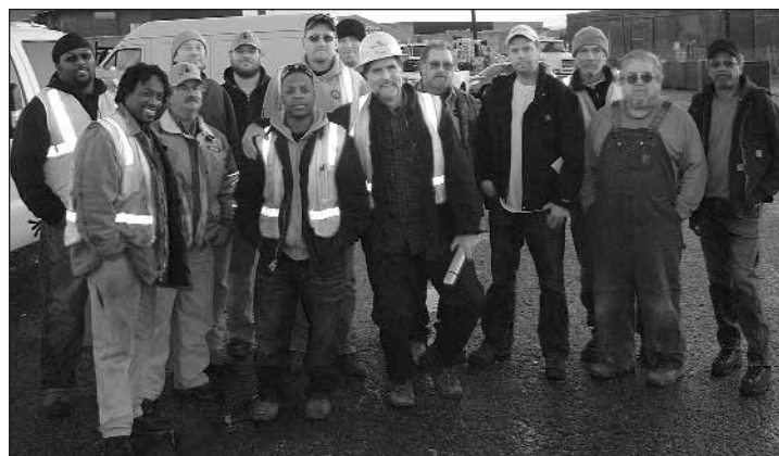
Picture of the Black & Veatch crew work on the final phase of the 115kv cable project between Hunter's point and Martin sub. These guys are pulling the cable in and splicing the cable in the conduit the Underground Construction installed early this year.
