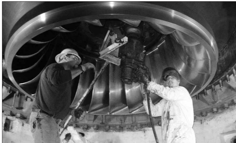
Senior Hydro Operator Dwayne Littlefield, left, and Plant Mechanic Jeff Fuller work on removing the turbine runner at Unit 2.
