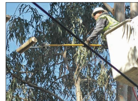
Foreman Eduardo Franco does some minor trimming from the bucket.
