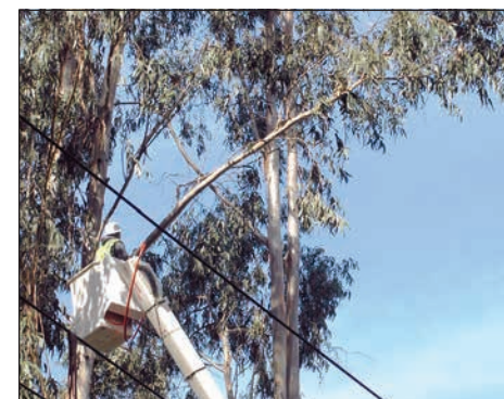
Branches leaning over like this pose a significant risk of falling into power lines during a storm.
