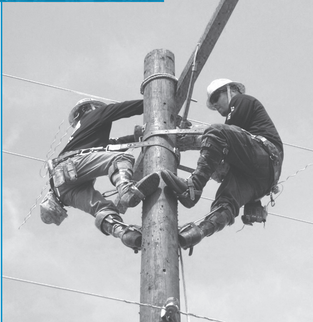
Branden Carter & Chris Fukui compete in the Cross Arm Change Out for SMUD. Photo by Crystal Candelaria
