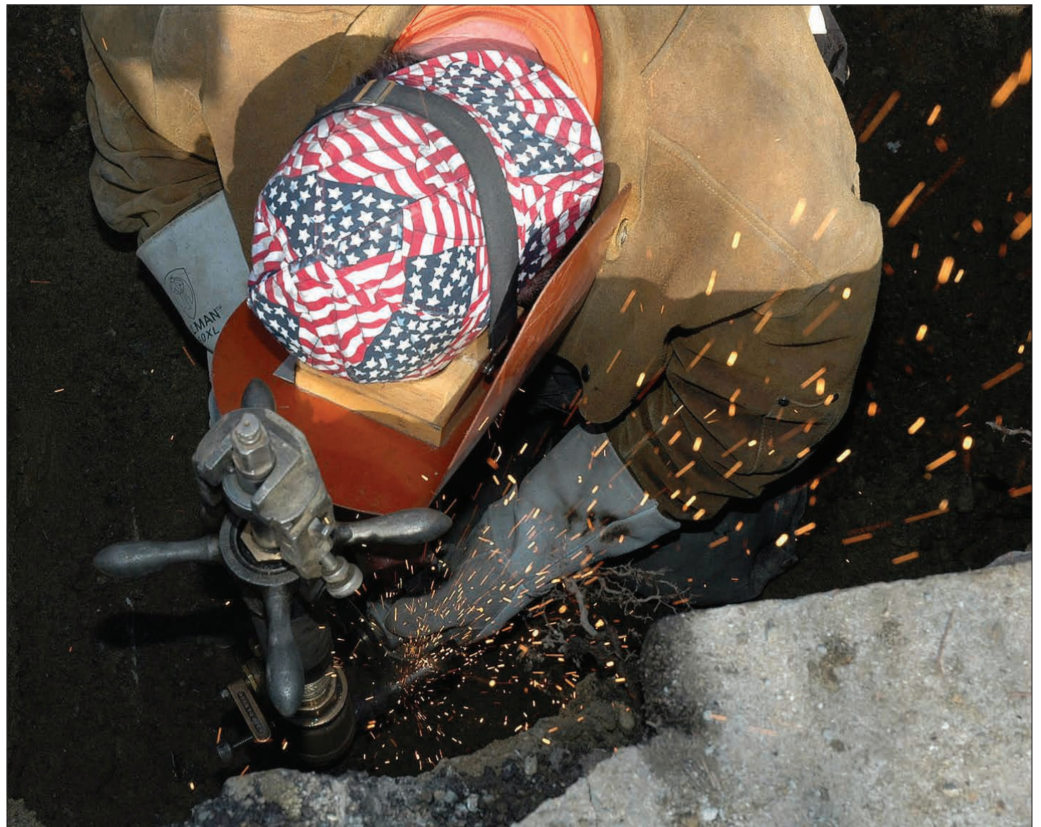
Neil Fuller welds the fitting.
