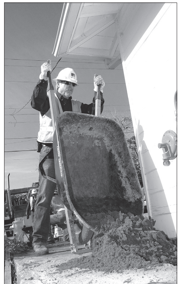
Tom Blum backfills the hole as the job wraps up.
