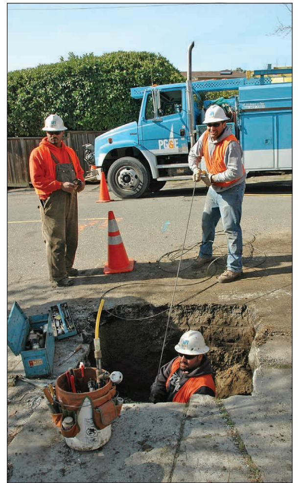
Joe Stringfellow (in the hole) and Alan Colaso: pulling.
