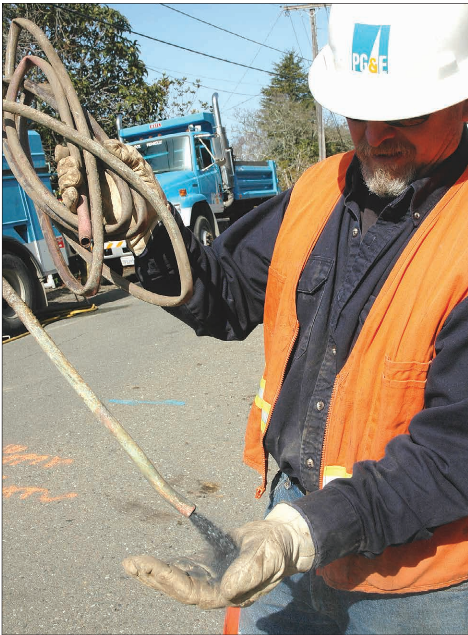
Tom Blum shows the flakey evidence of corrosion in the copper pipe.
