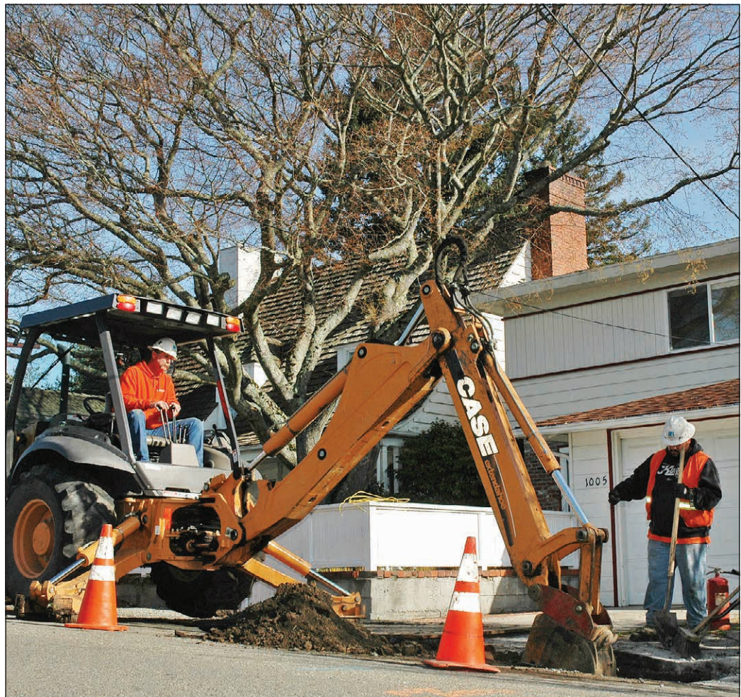
Backhoe Operator Larry Lee digs down to the Service-T.
