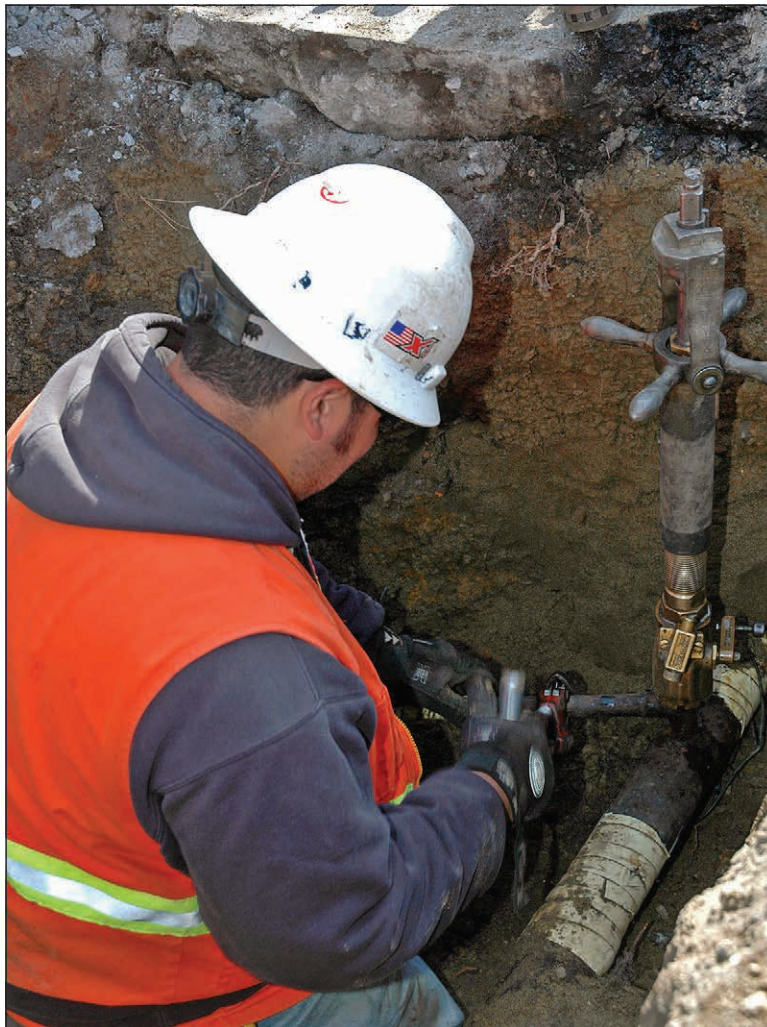
Joe Stringfellow stops the flow of gas to service and prepares for the welder.
