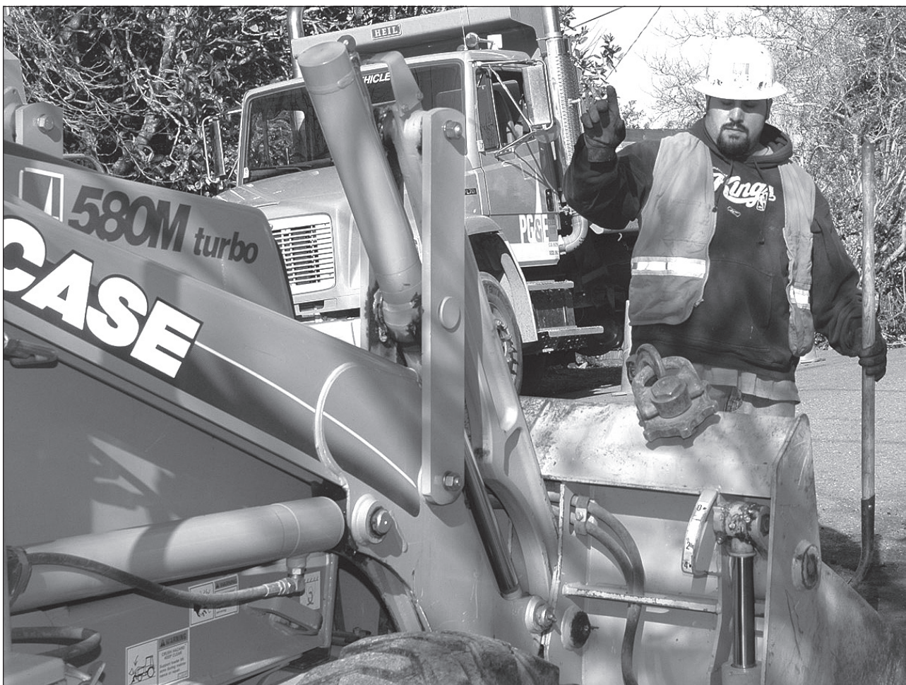
Joe Stringfellow signals the backhoe operator.
