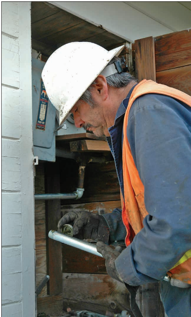
Ramon Moreno works on installing the gas meter in its new location—outside the electric box.
