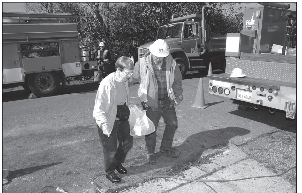
Working Foreman Kirk Cardoza assists a resident through the construction area.
