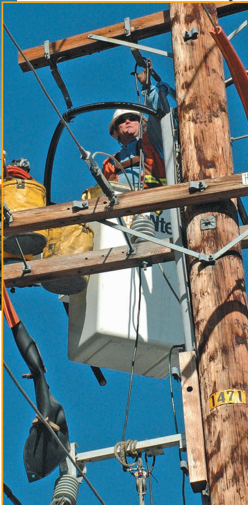
Skip Alcorn relocates a temporary protective grounding cable in order to land the new 1100 Al cable at top of riser pole.
