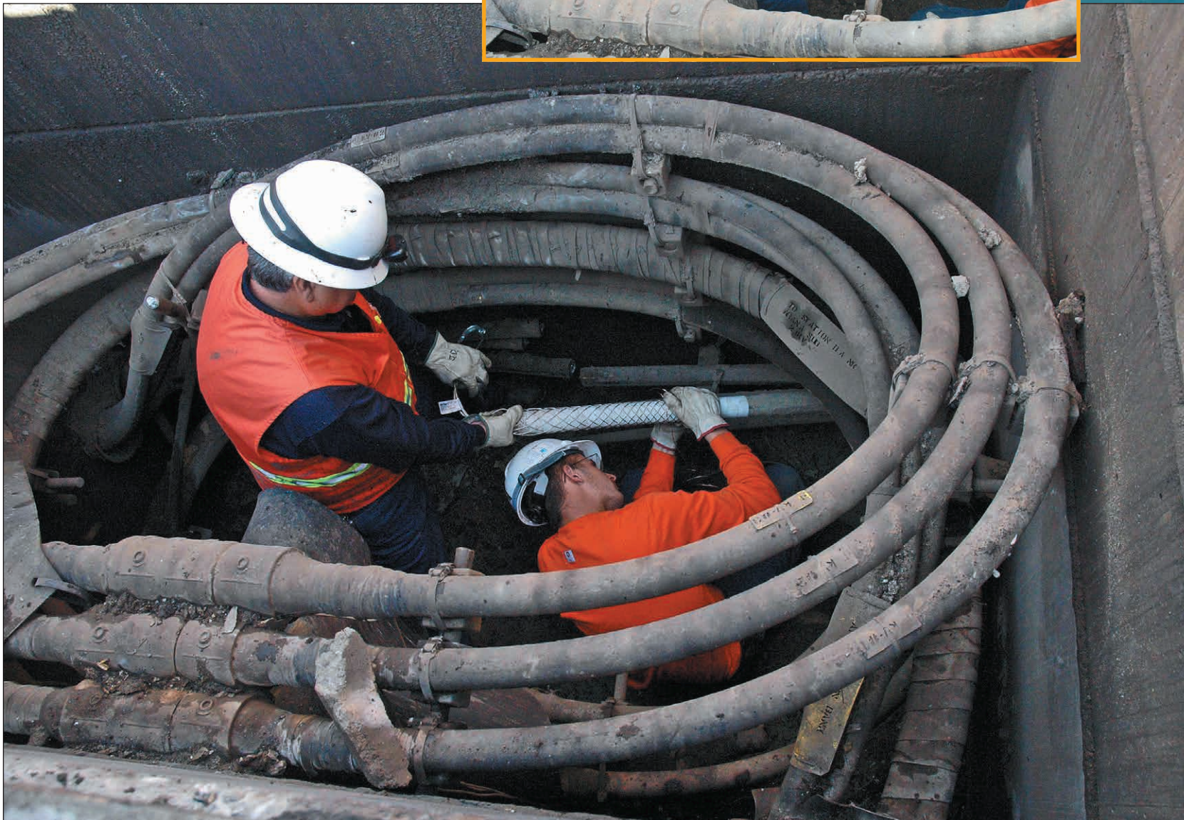
Mike Farinsky, Jr. secures a Kellum grip on to a cable in order to pull in braided rope on Soquel Avenue in Santa Cruz. Working in the vault with him is J.D. Sotelo.
