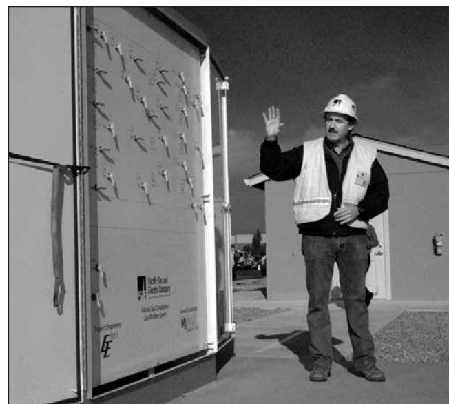
Luis Faria, a Senior Instructor at San Ramon, shows off the master panel that controls gas flow to various training center locations.
