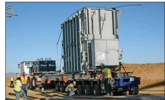
Operators slowly back the transformer onto the pad.
