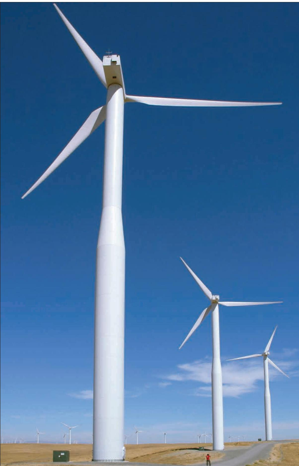
Phase 2 wind turbines at SMUD's Solano Wind Project stand 415 feet high. The rotor diameter is 295 feet—about the length of a football field.
