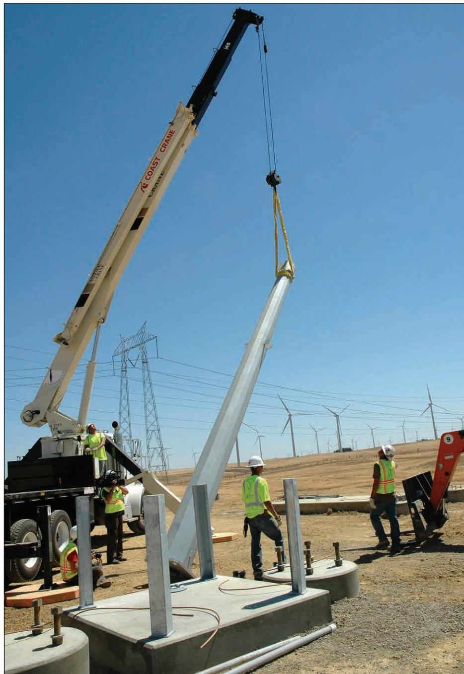
Crane Operator Greg Ekwall of Rosendin Electric (at left) hauls steel into place in late September for the new substation at the Shiloh II wind project.
