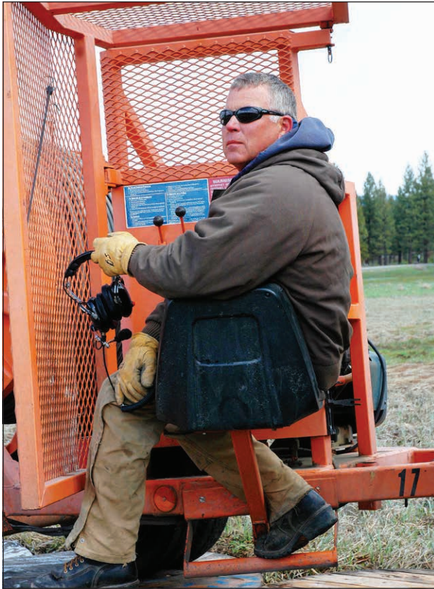
Lineman Bruce Smith, shown here at the controls of the tensioner, is a union steward and serves on the union bargaining committee.
