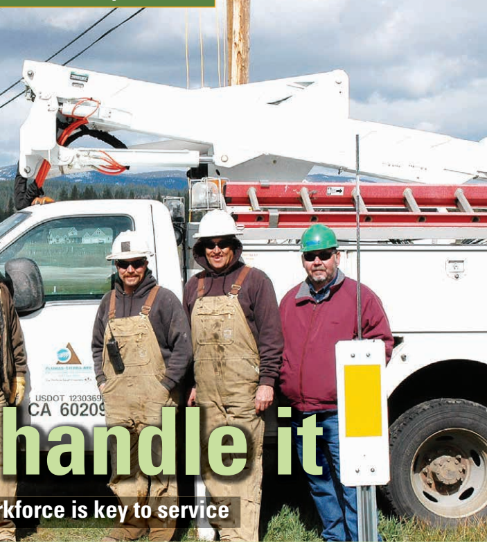
(LEFT) Working the reconductoring job along Highway 89 are, from left: Linemen Nathan Norton and Mitchell Carr, Troubleman Greg Goodrich, Lineman Bruce Smith, Foreman Paul Erwin, and Lineman Guy Varner. Joining them for the photo is Local 1245 Business Rep. Randy Osborn.
