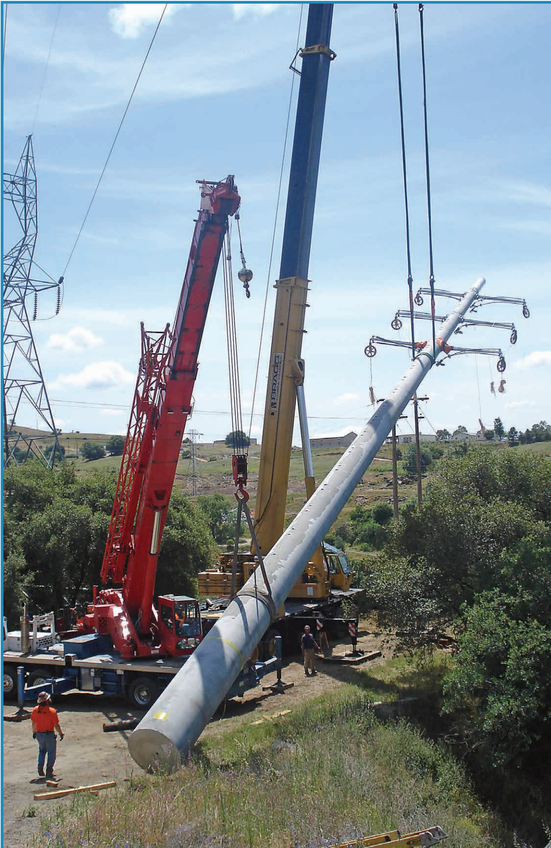
SMUD crew (above) installs a steel transmission pole in two pieces. Poles weighing between 40 and 70 thousand pounds are hefted into position (below and right).
