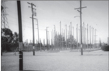
PG&E's San Ramon Learning Center (top) and Livermore Training Center drew high praise from Joe Carl, IBEW's Regional Training Coordinator. "What you have at PG&E is ... state of the art—the infrastructure, instructors, relation to Local 1245. It's awesome." Photos: Larry Pierce
