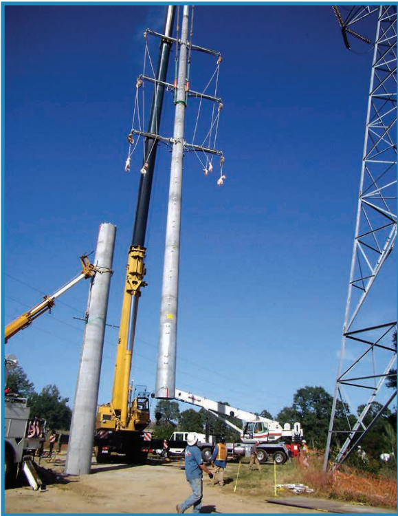
SMUD crew (above) installs a steel transmission pole in two pieces. Poles weighing between 40 and 70 thousand pounds are hefted into position (below and right).
