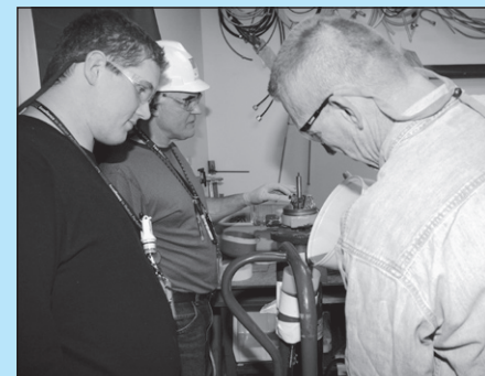
Emergency diesel generators provide back-up power for the emergency cooling pumps. Working on a switch calibration are Nic Evangelo, Apprentice Instrument Repairman; Jim Bennett, Shift Control Technician; and Mike Symens, Apprentice Instrument Repairman.
