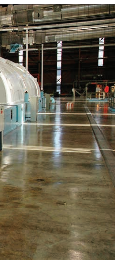
The turbines are what Diablo Canyon is ultimately about, utilizing steam heated by a nuclear reaction to generate electricity. Business Rep. Dan Lockwood stands in the cavernous room where the action is.
