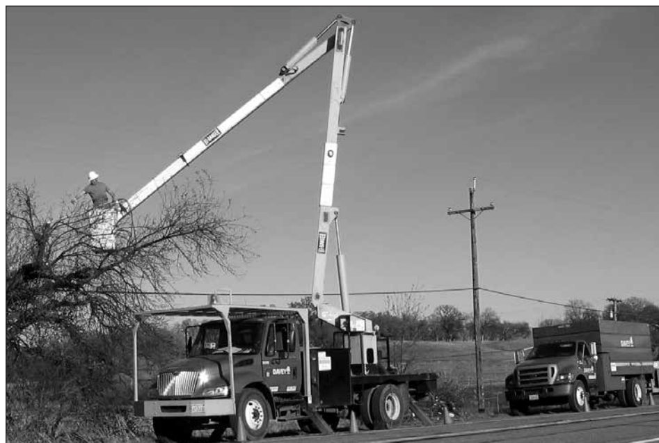
A Davey Tree crew performs line clearance tree trimming just east of Dry Creek on Highway 299 in California. In the lift is Working Foreman Gil Suarez, a 12-year member of IBEW Local 1245. Also working on the job, but not pictured, is Climber Travis Payton, initiated in 2004.
