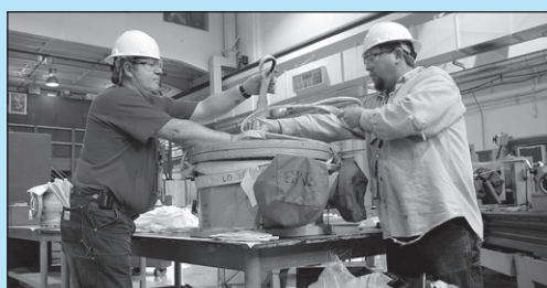
Mechanic-Riggers Robert Turney, left, and Al Etchison prepare to move a channel head for a heat exchanger on a diesel generator.
