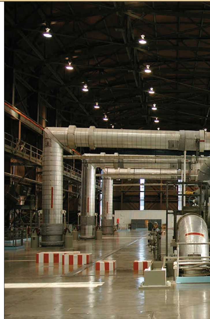
The Unit 2 turbine, on the 140' level of the "Turbine Deck."
