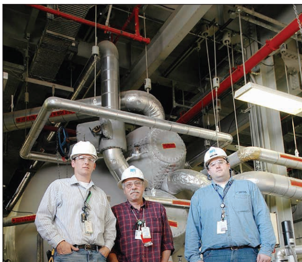
Standing in front of the moisture separators are Operators, from left, Frank Eric Lowe, John Clipperton and Jack Kiser.
