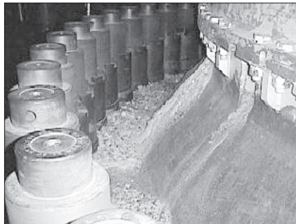
Red rusty boric acid deposits on the Davis-Besse vessel flange. NIRS.org
