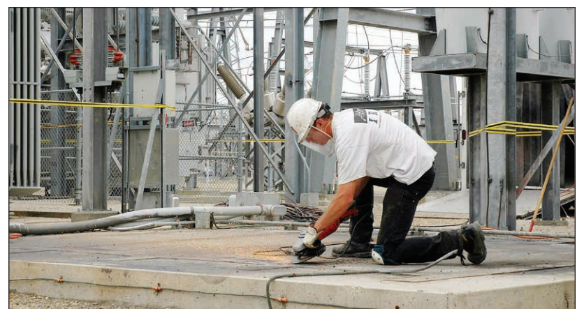
IRH/ABN employee is grinding smooth the surface where the transformer was cut loose from the pad.
