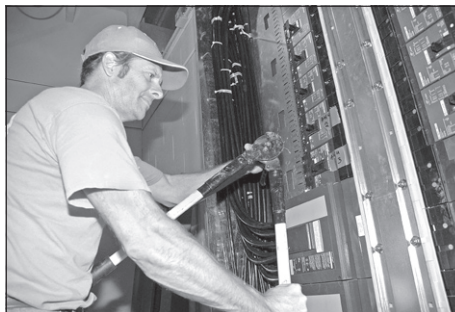
Jeffrey Johnson at work. IBEW Local 130 now has 1100 members serving the New Orleans area, about the same number as before Katrina.
