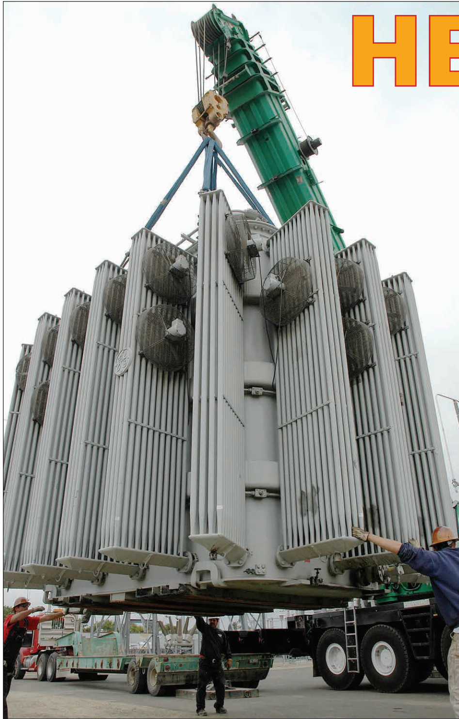
IRH/ABN crew moves a transformer that is about to be cut up for salvage.
