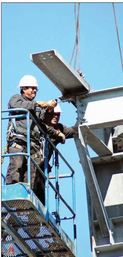
A wrench is used in dismantling part of the tower structure.
