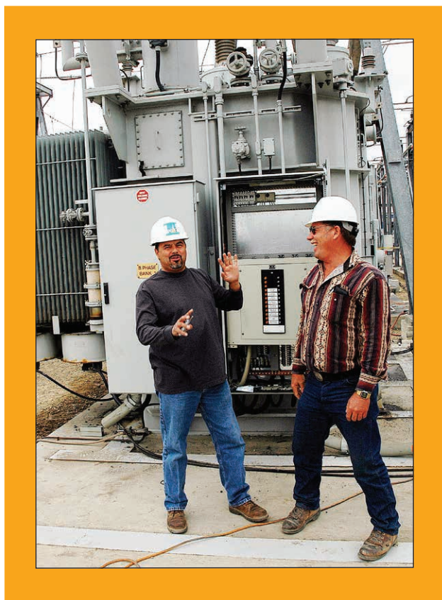
PG&E Electric Tech Gary Henry, left, and Working Foreman B Jim Bradley share a lighter moment at the East Shore Substation.
