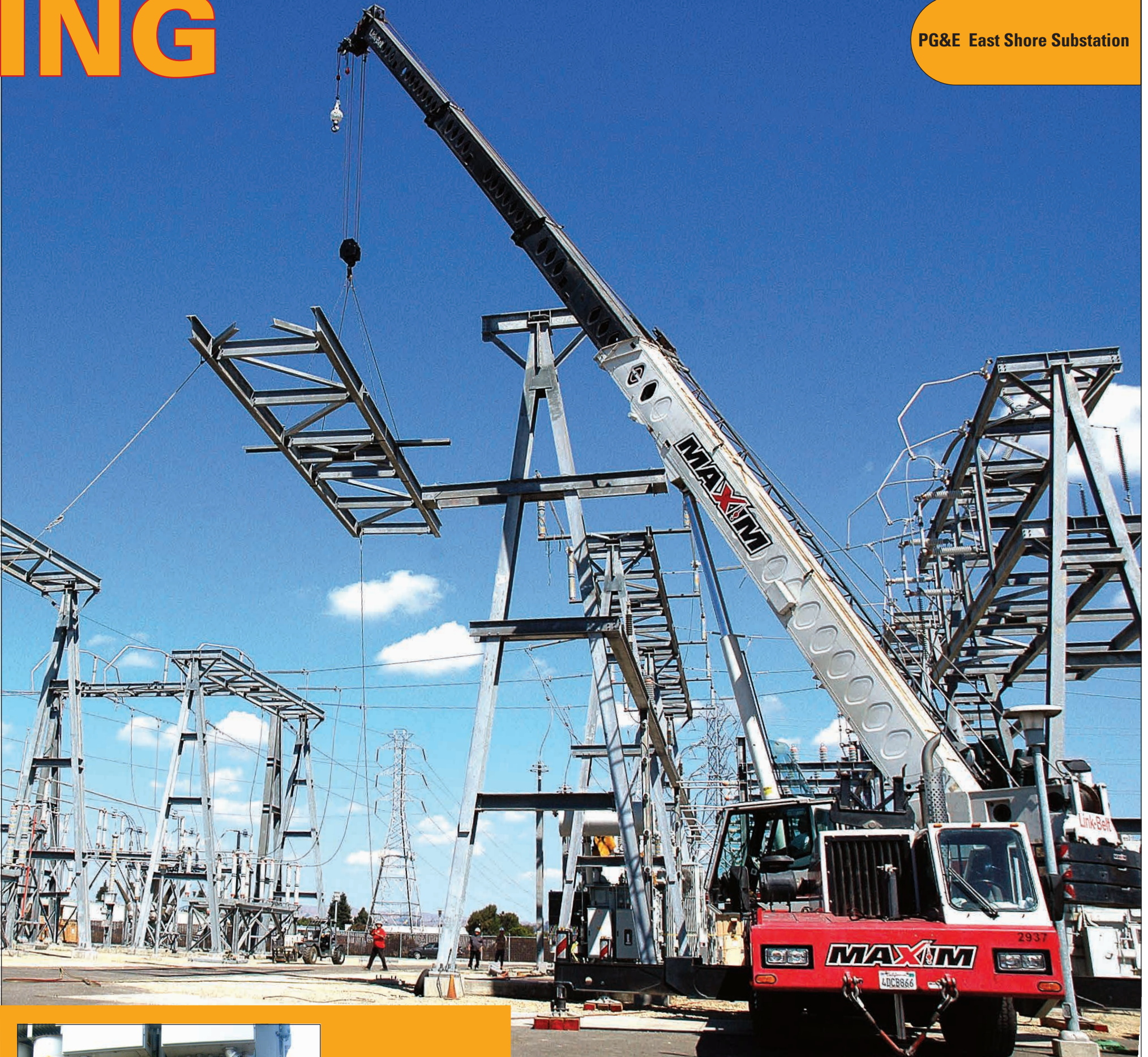
After being cut free from the tower, the “bridge” is carefully lowered to the ground.
