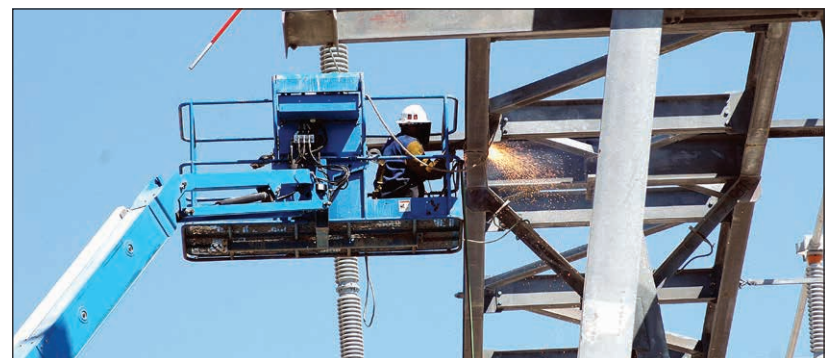
Using a torch to cut a beam from the tower structure so that it can be removed.
