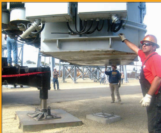
The transformer is being relocated so IRH/ABN can cut it up for salvage.
