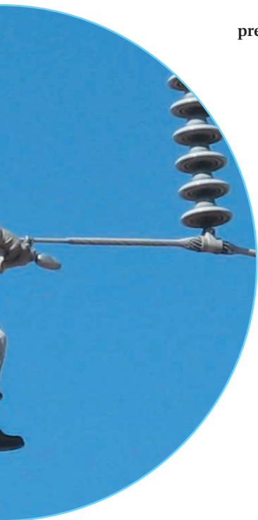
BELOW: Russ Rylee on left holds on the energized conductor while Joe Ferreira installs vibration damper.
