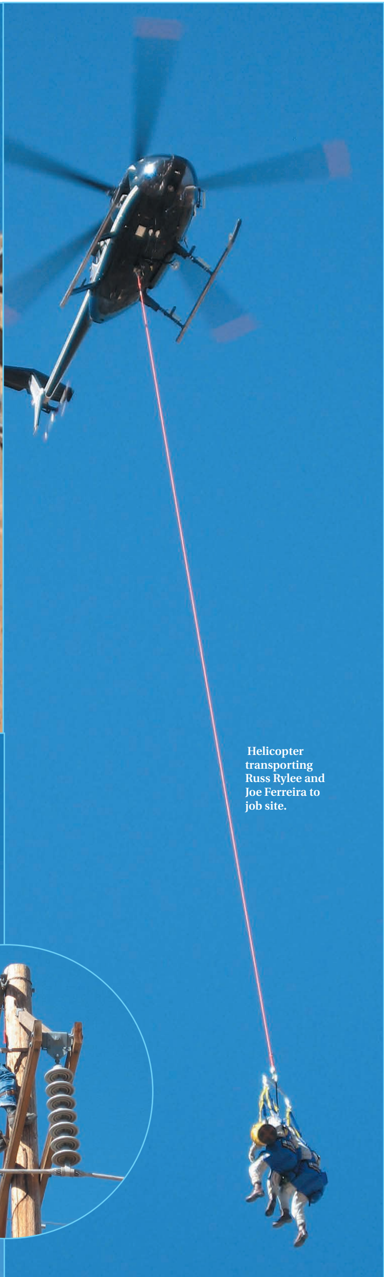
Jim McAdams GC lineman demonstrating PG&E's long line pole transfer.
