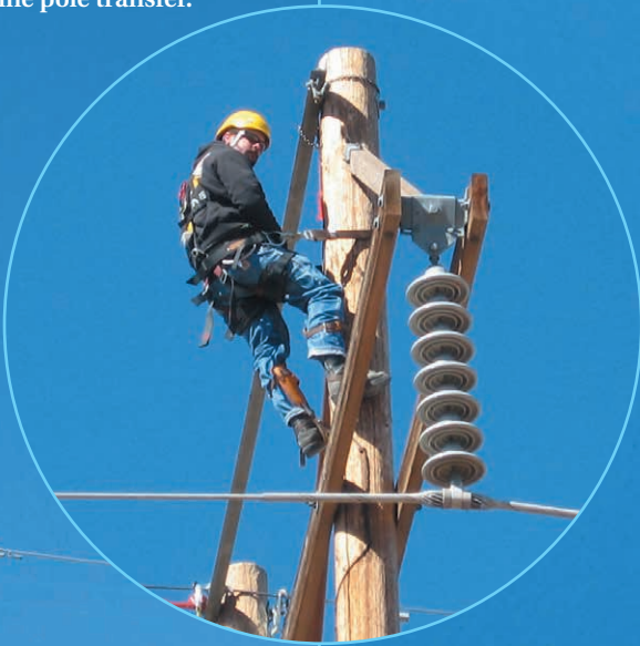
Jim McAdams GC lineman demonstrating PG&E's long line pole transfer.
