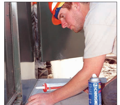
Groundman Michael Stover applies caulk to the transformer.
