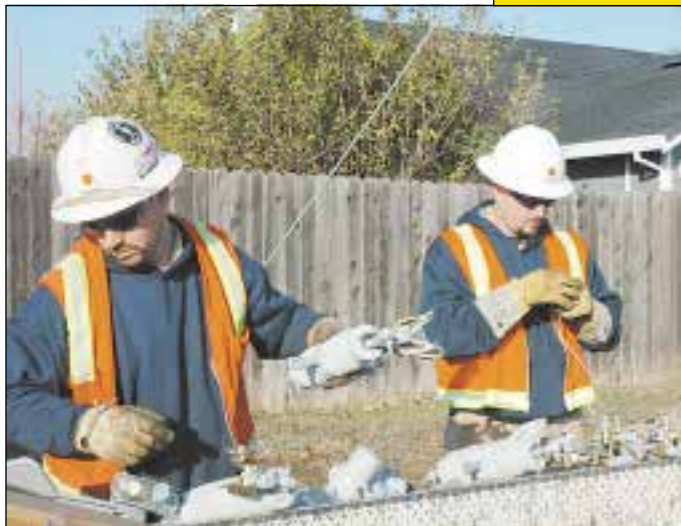
Preapprentices Tom Jasper, left, and Eric Dixon prepare the equipment needed for the job.
