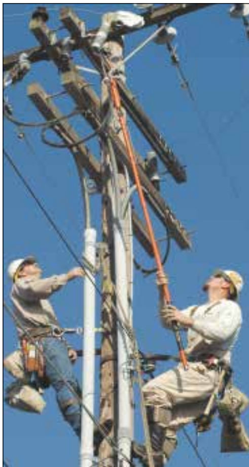
Lineman Frank Cotter observes as Apprentice Corey Smith prepares to close the cutout with a shotgun.
