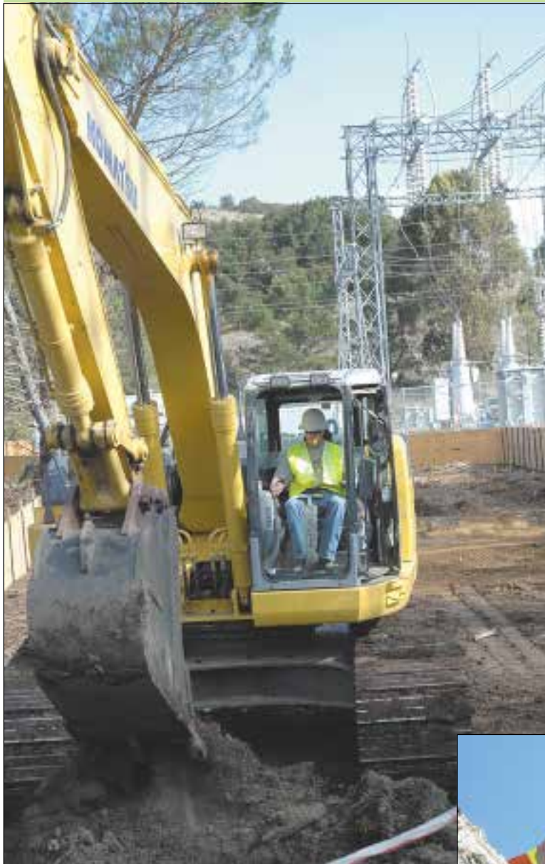
Todd Francis operates the backhoe. Jefferson Substation is in the background.
