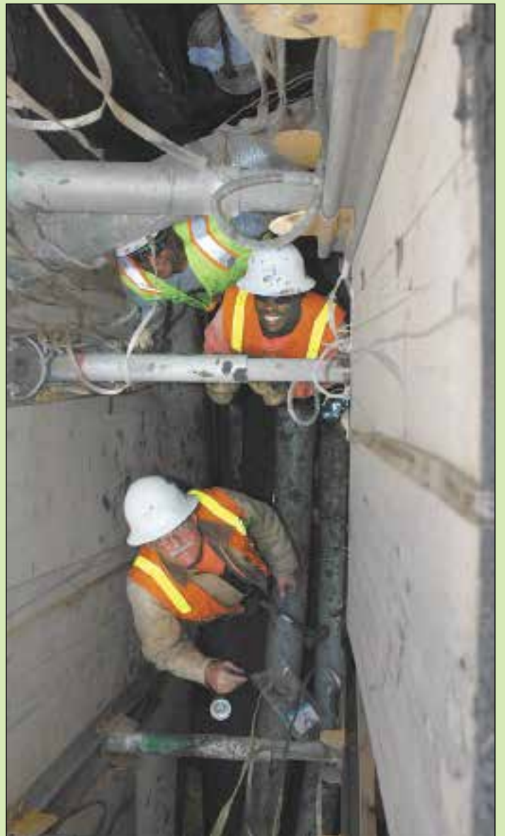
Working the conduit deep in the trench are, from top to bottom, Groundmen Jacques Johnson and Treobia Battles, and Operator Patrick Wynkoop.
