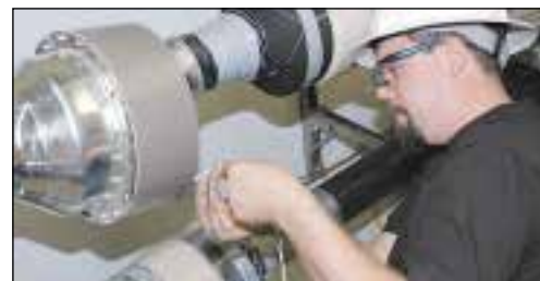
Lineman William Kessel: "If protection were to fail, it could explode like a bomb."
