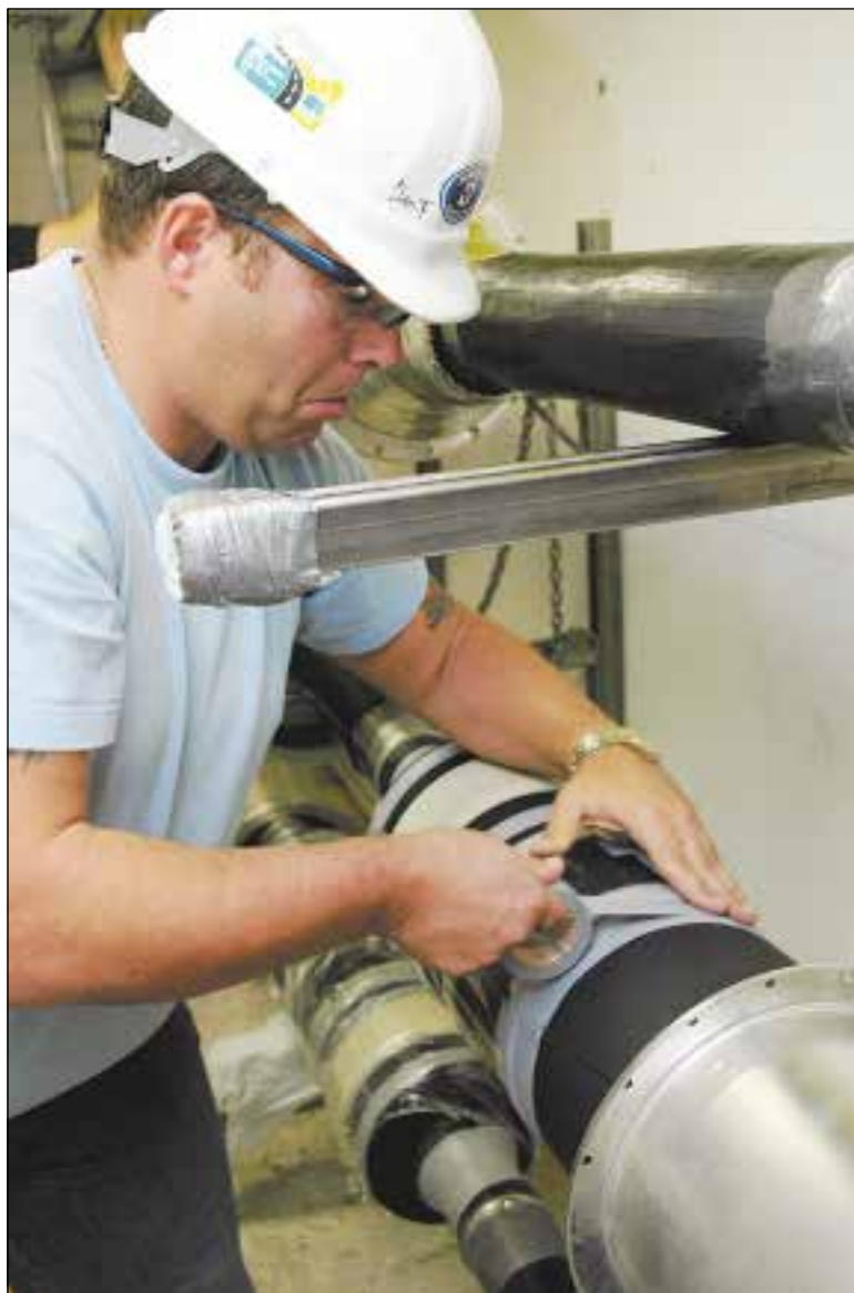
Cable Splicer Jan Flipse tapes a joint.
