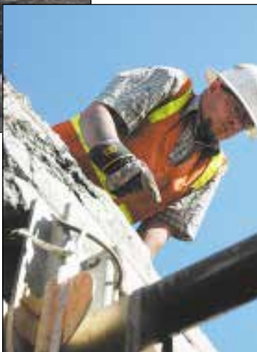
Groundman George Marshall remains above, ready to lower down whatever is needed in the trench.
