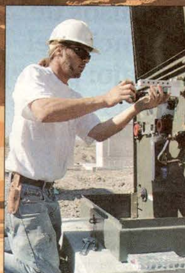
Sam Green hooking up the hardware in the pad mount transformer.
