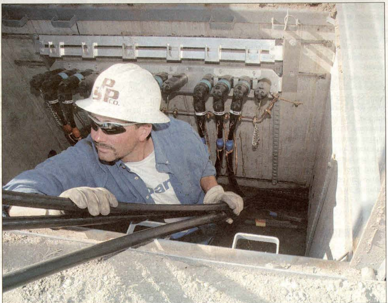
BELOW: Lineman Wade Henderson ignores the water at his feet as he helps pull the cable into the vault for its journey through the underground.
