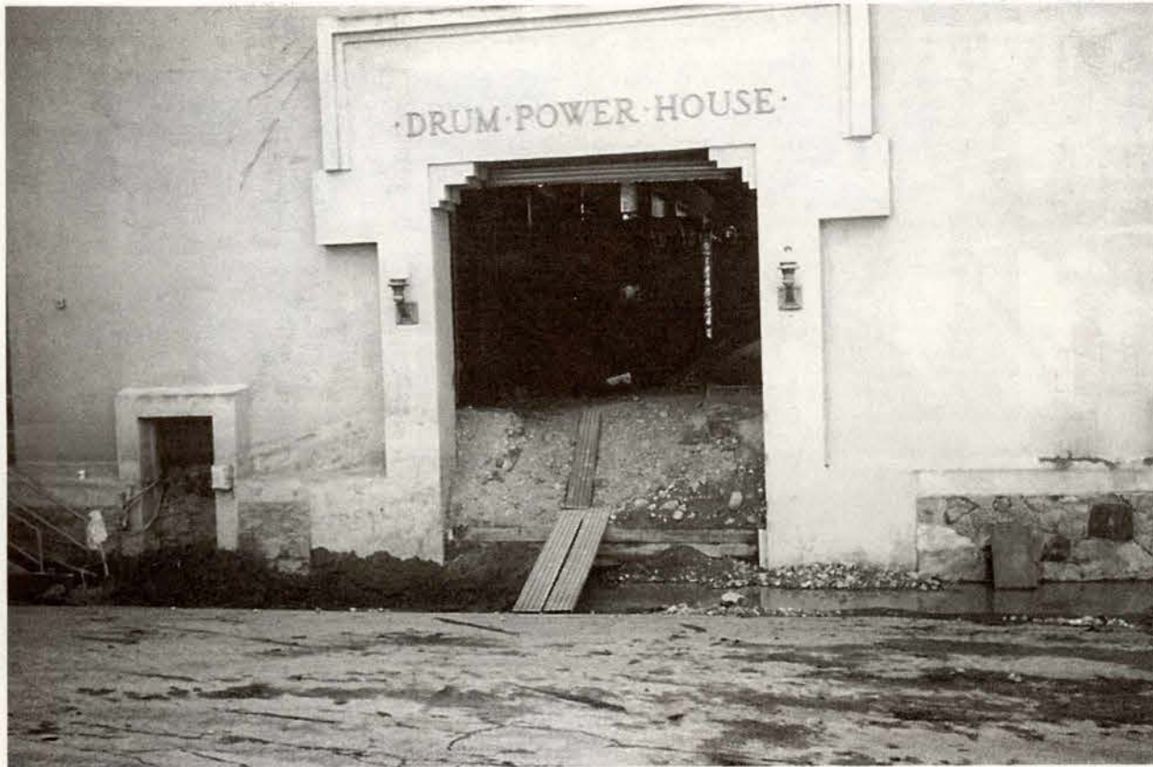
400,000 cubic yards of dirt were hauled out of the power house and afterbay.
