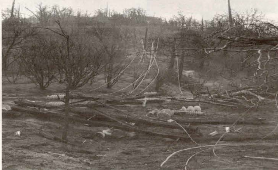
Electric facilities in southern California were devastated by six major fires. In the San Diego area alone, crews worked to set approximately 1500 poles, replace 1.5 million feet of overhead wire, and rebuild 17 major transmission facilities.
