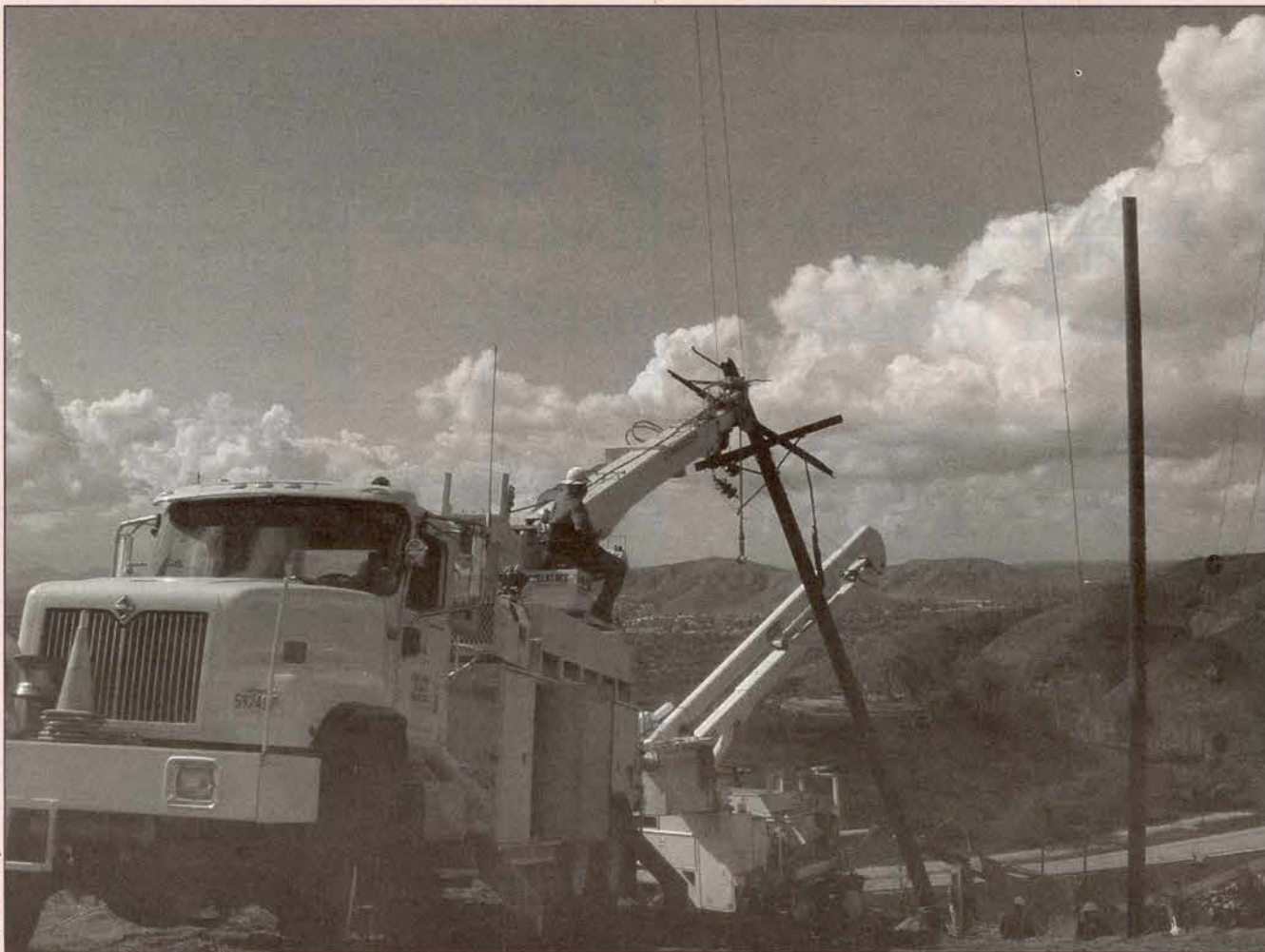
Sierra Pacific Power crew setting new poles in an area devastated by the fire.
