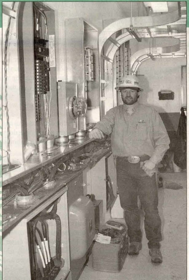
Fourth-year Apprentice Electrician Kevin Vial, a 10-year IBEW member, shows off the progress made on the new building.
