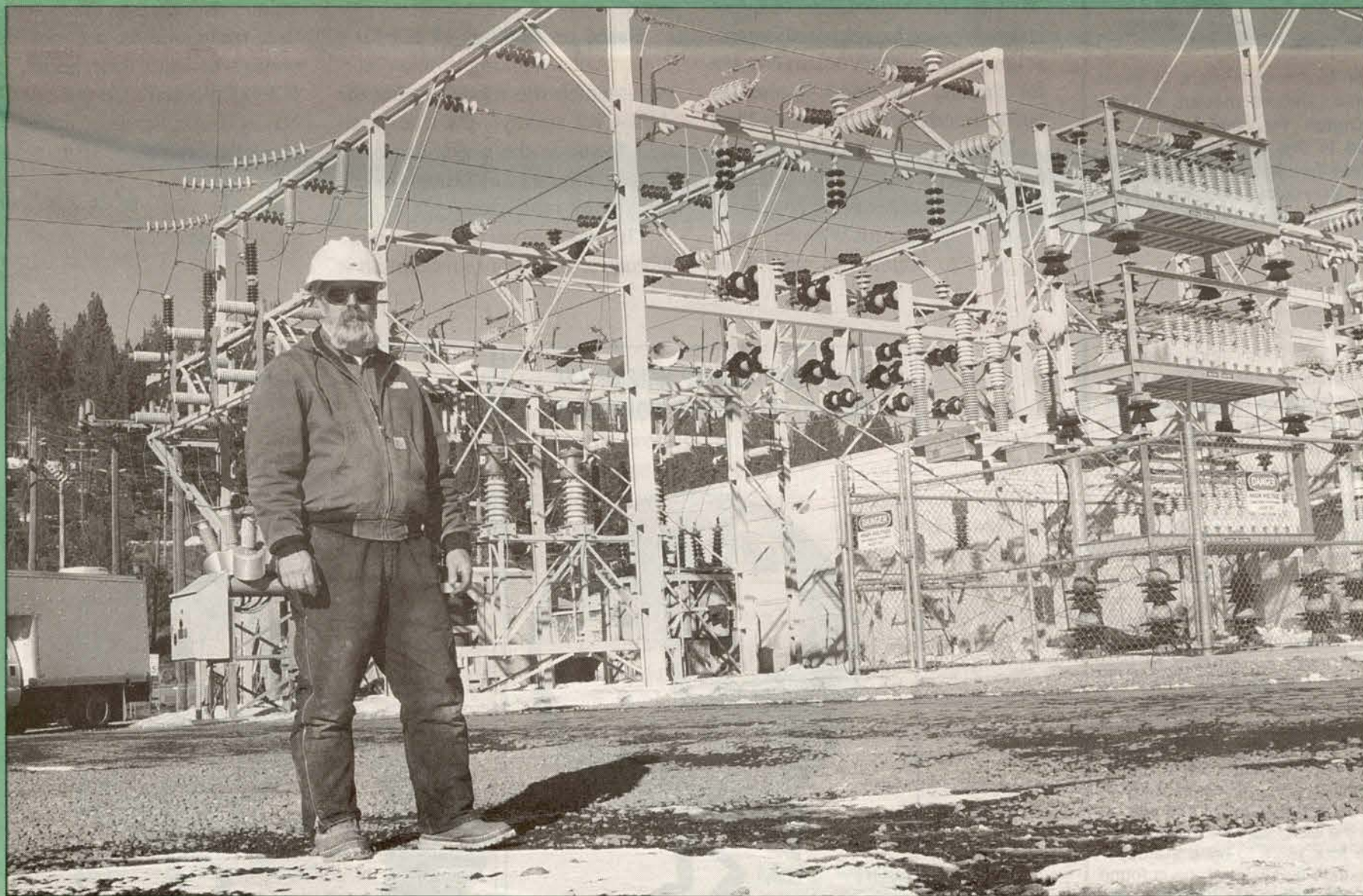
Control Foreman Mike Coli, a 23-year IBEW member.
