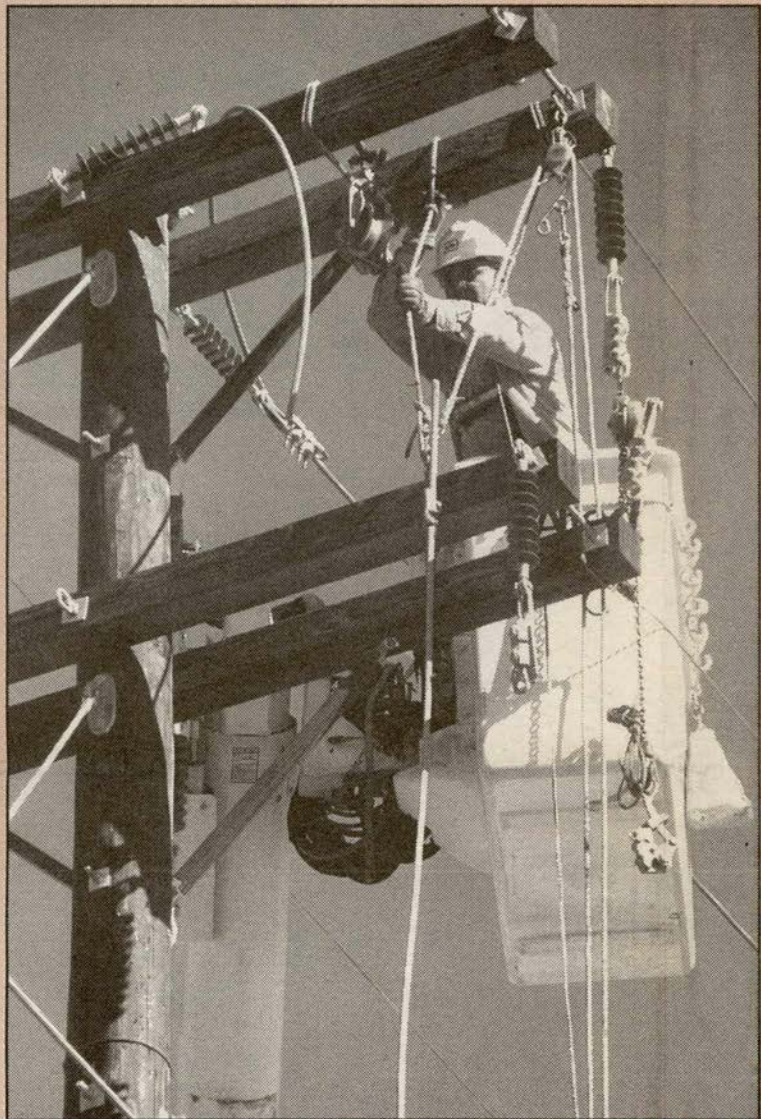
Barry Mitchell, lineman for Harker & Harker, a contractor assisting on the job.
