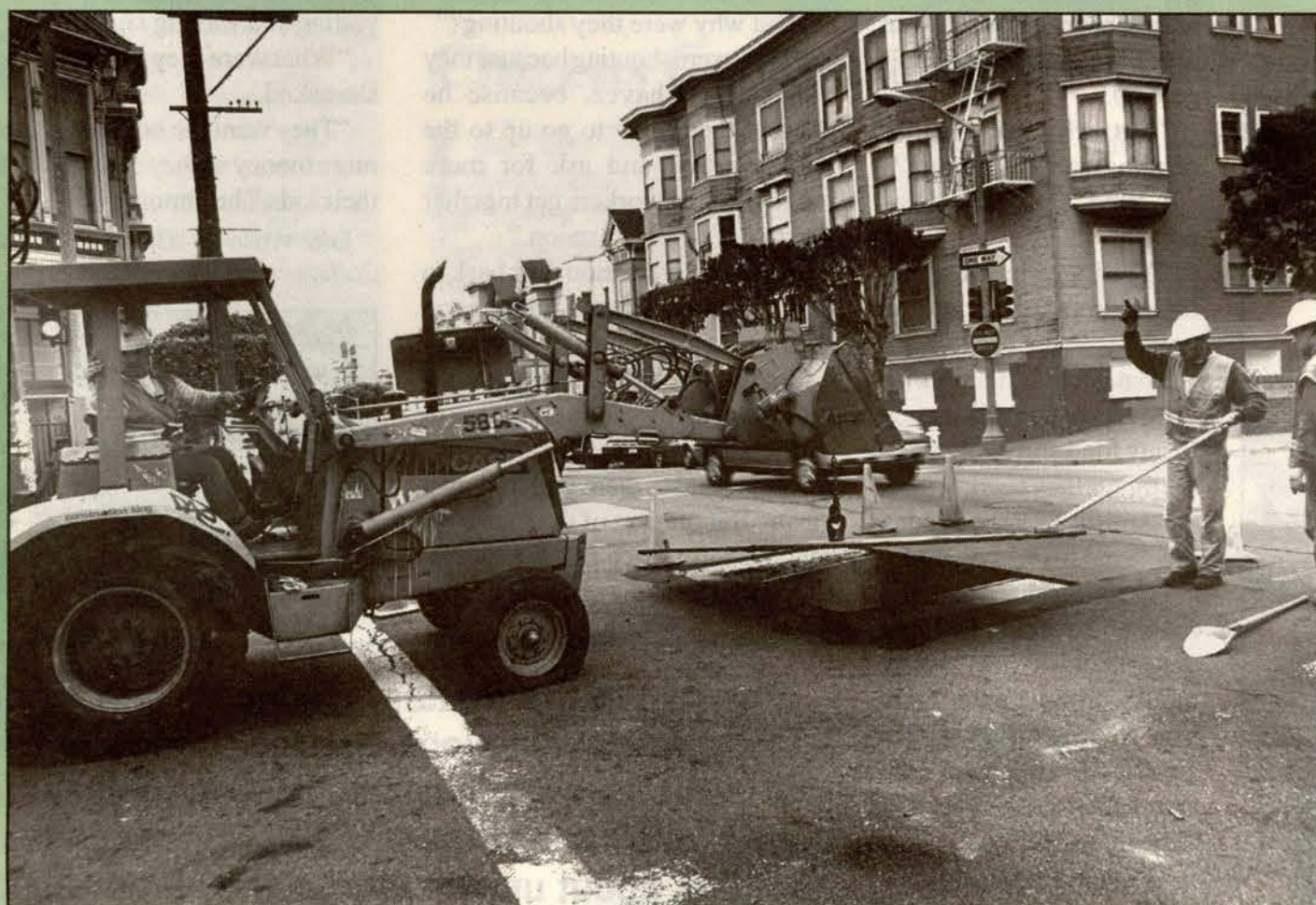
Jose Castellanos, mechanical equipment operator; Ross Ortega, fieldman; Ken Lowther, utility worker
