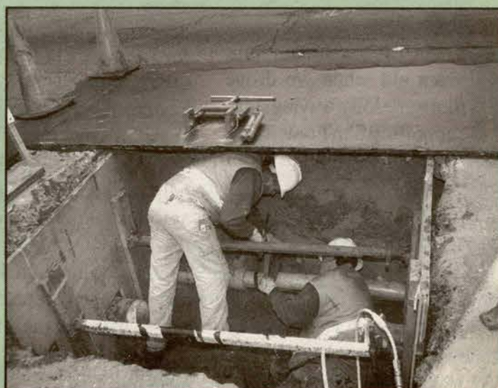
Ross Ortega, fieldman; Ken Lowther, utility worker
