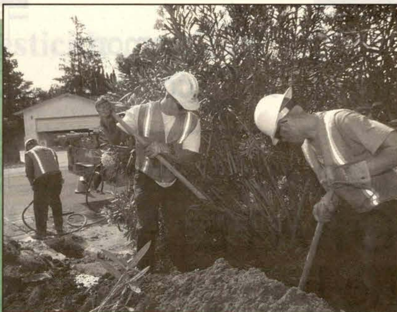
This Sacramento Municipal Utility District crew installing a residential service in a northeastern Sacramento neighborhood consisted of Lucas Raley and Greg Baird, apprentice linemen, and Garry Dremel, upgraded light foreman.
