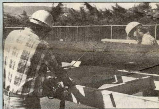
Sierra Pacific maintenance crew in a routine job: loading a pole up in the yard for transport to the Mt. Rose substation, where a hole will be re-dug and the pole set. (Photos: Eric Wolfe)
