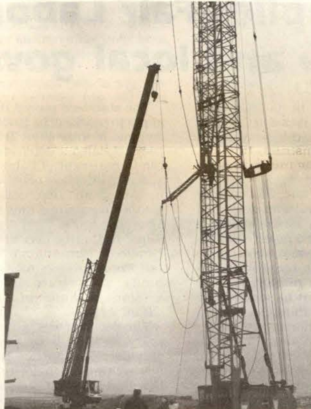
Small crane sets up large tower crane.
